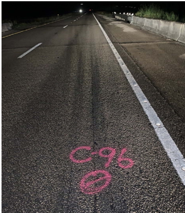
Partial Core Unable to fully extract core from bridge deck.
