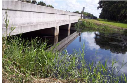
East side of bridge.
