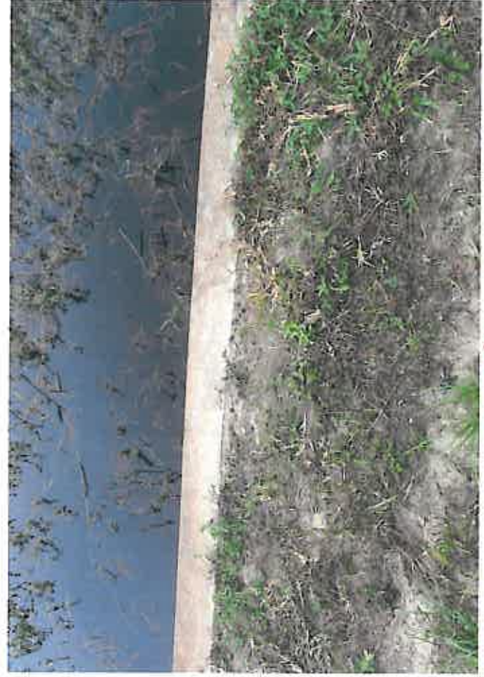
SR 29 Cross Drains (mp 5.50 and 6.257) Glades
