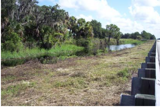
Ditch on northwest side of bridge.
