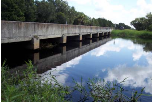
East side of bridge.
