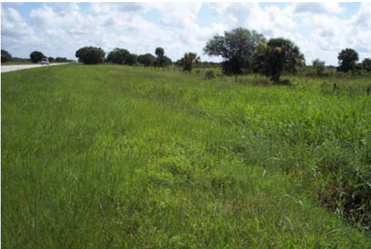
Ditch on northeast side of cross drain.
