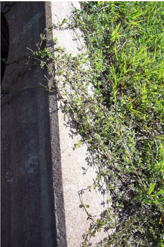
Headwall on west side of cross drain.
