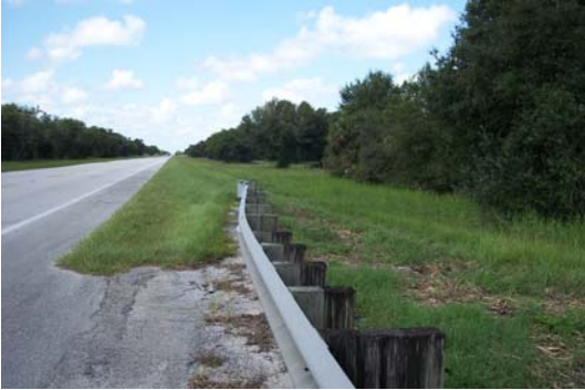
Ditch on southwest side of bridge.
