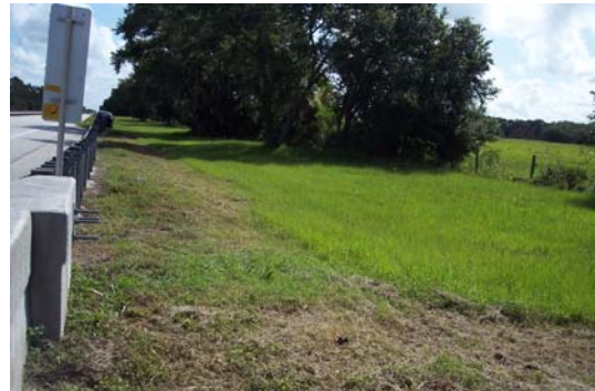
Ditch on northeast side of bridge.
