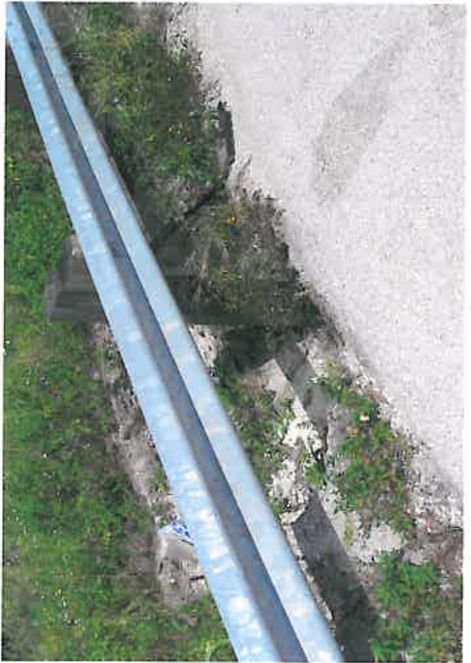
SE29 Cross drain
