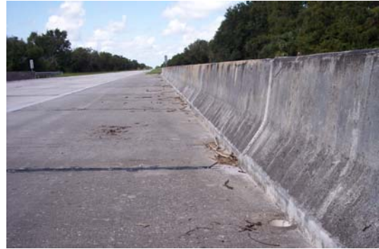
Facing south along shoulder, west side of bridge.
