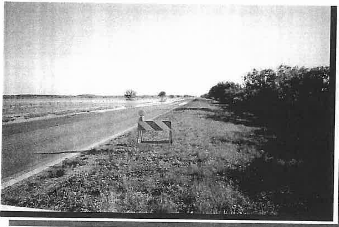
LOOKING NORTHEAST ALONG S.R. 29 BETWEEN LONE PINE CREEK AND CHAPARRAL SLOUGH
