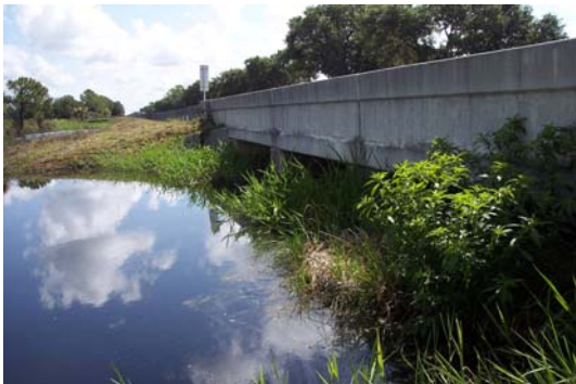
West side of bridge.
