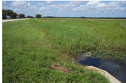
Ditch on southwest side of cross drain.
