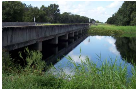
West side of bridge.
