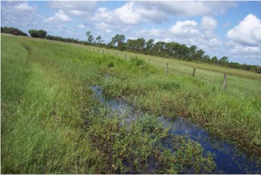
Ditch on southwest side of cross drain.
