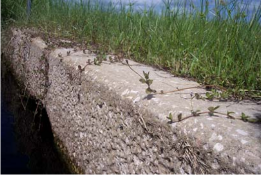
Headwall on east side of cross drain.
