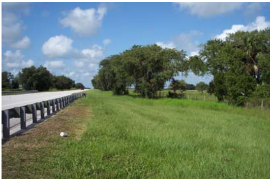
Ditch on southwest side of bridge.
