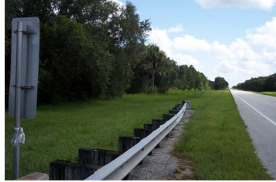
Ditch on northwest side of bridge.
