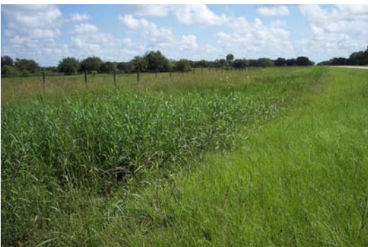
Ditch on northwest side of cross drain.
