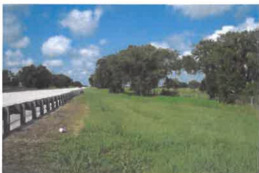
Ditch on southwest side of bridge.
