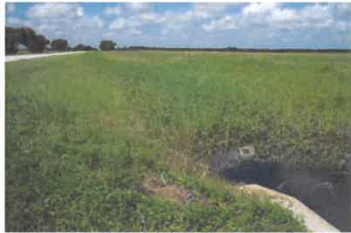
Ditch on southwest side of cross drain.
