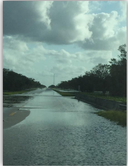
Figure 11: Hurricane Irma (2017) SR 29 Flooding Photo 2
