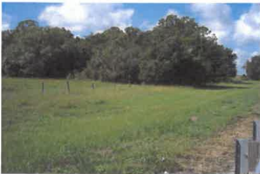
Ditch on southeast side of bridge.
