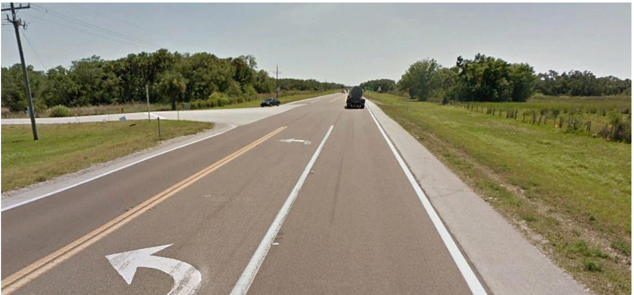
SR 29 Southbound View
