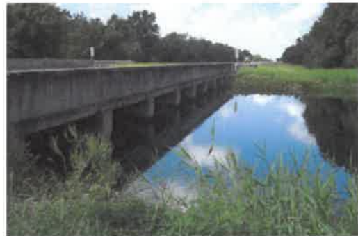
West side of bridge.
