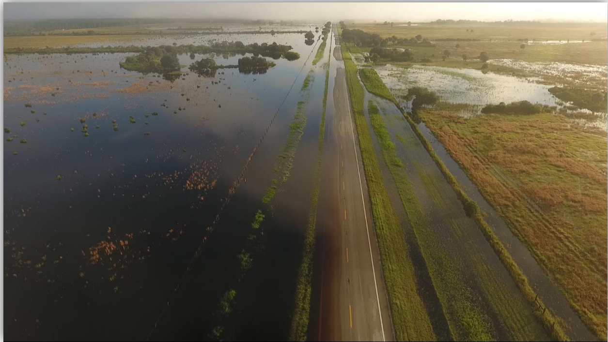
Figure 13: SR 29 Flooding September 22, 2021 Photo 2
