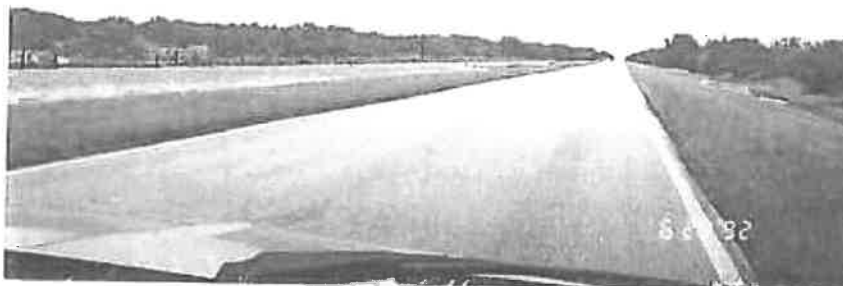
SR 29 - Between Bridge 050033 and SR 78 on June 29, 1992 - wet season.
