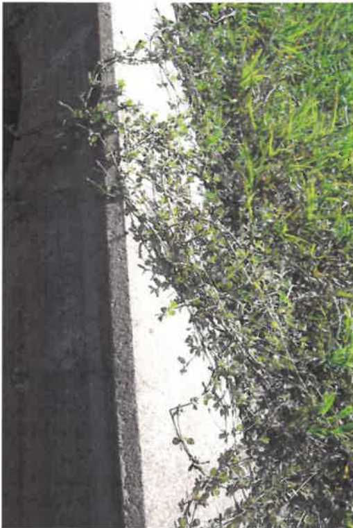
Headwall on west side of cross drain.
