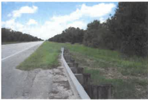
Ditch on southwest side of bridge.
