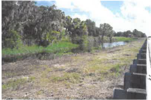
Ditch on northwest side of bridge.
