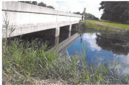
East side of bridge.
