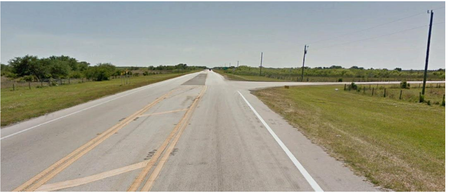
SR 29 Southbound View
