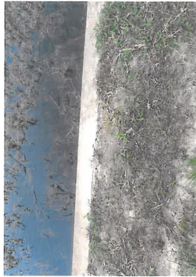
SR 29 Cross Drains (mp 5.50 and 6.257) Glades
