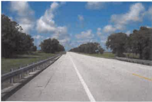
Looking south along S.R. 29 from the bridge culvert.
