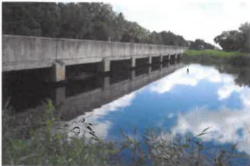
East side of bridge.
