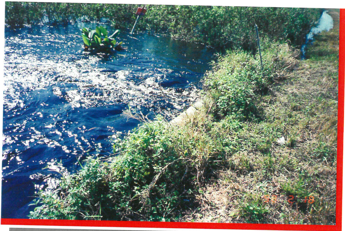
LOOKING SOUTH ALONG S.R. 29 AT (3) 30" RCP APPROXIMATELY STA. 354+00
