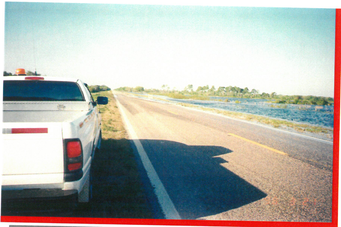
LOOKING SOUTHWEST ALONG S.R. 29 BETWEEN LONE PINE CREEK AND CHAPARRAL SLOUGH
