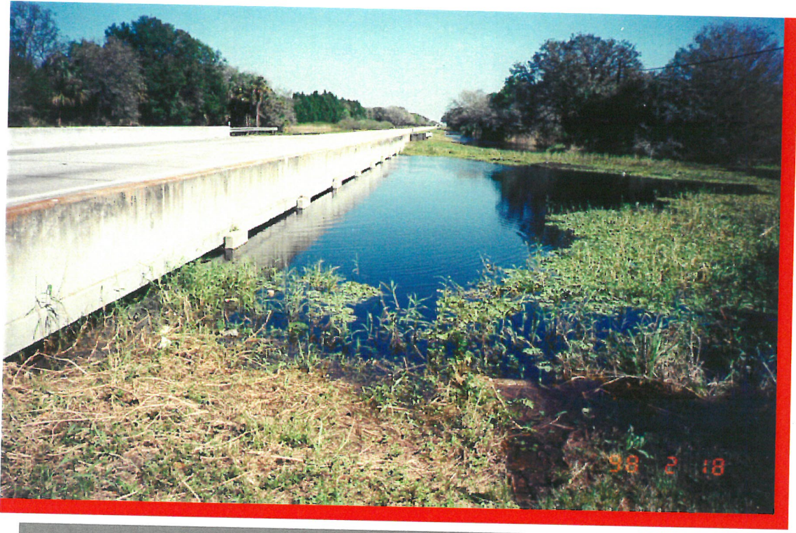
LOOKING NORTHEAST ALONG S.R. 29 AT CHAPARRAL SLOUGH BRIDGE
