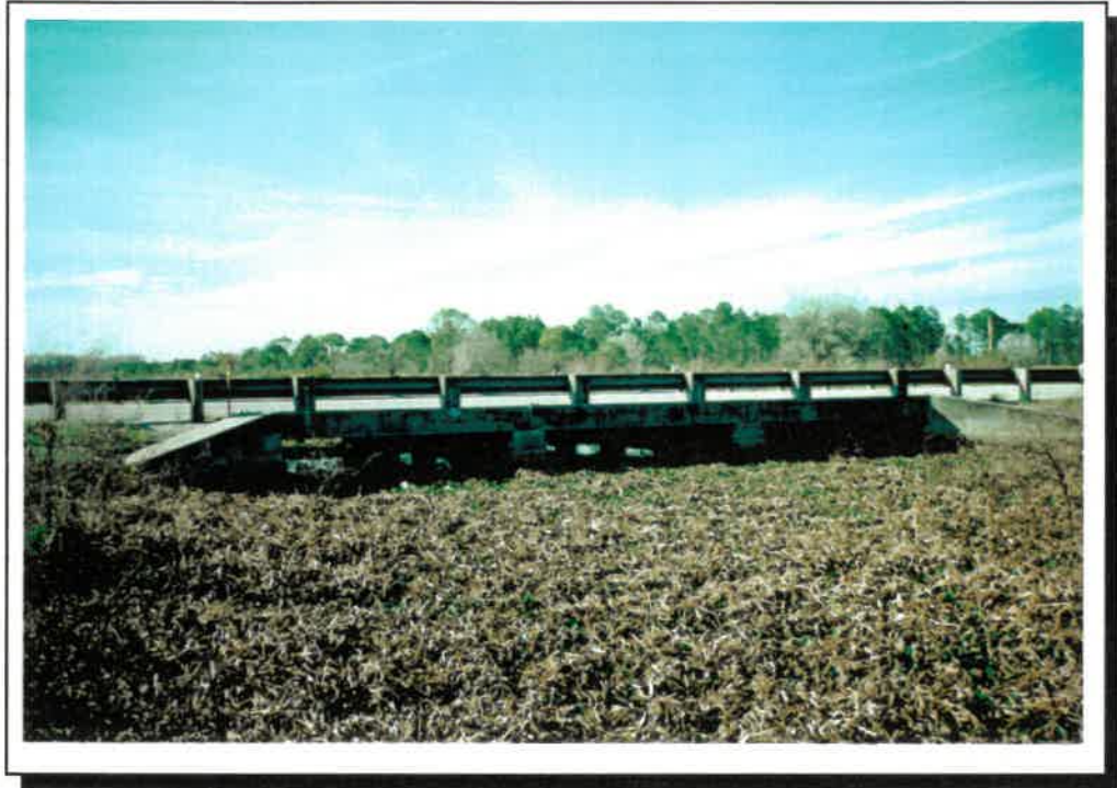
Bridge No. 050032: Upstream Elevation and Cover Shot
