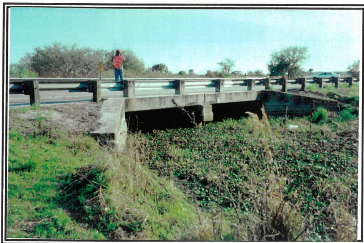
Figure A-2: Bridge No. 050031, Upstream Elevation
