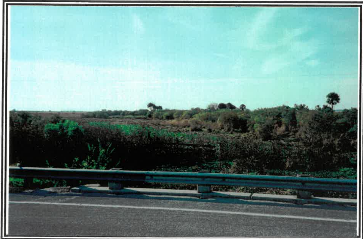
Figure A-4: Turkey Branch, View Upstream of SR 29 Bridge
