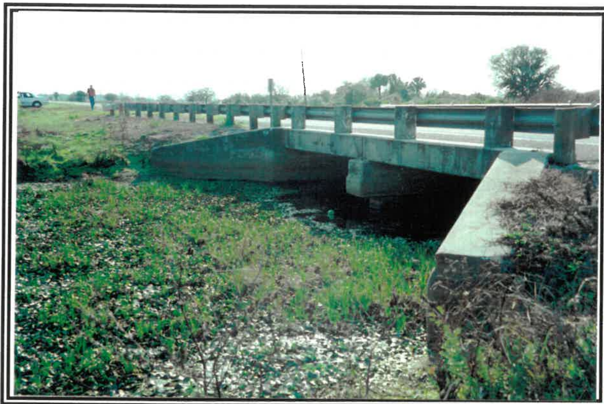
Figure A-1: Bridge No. 050031, Downstream Elevation
