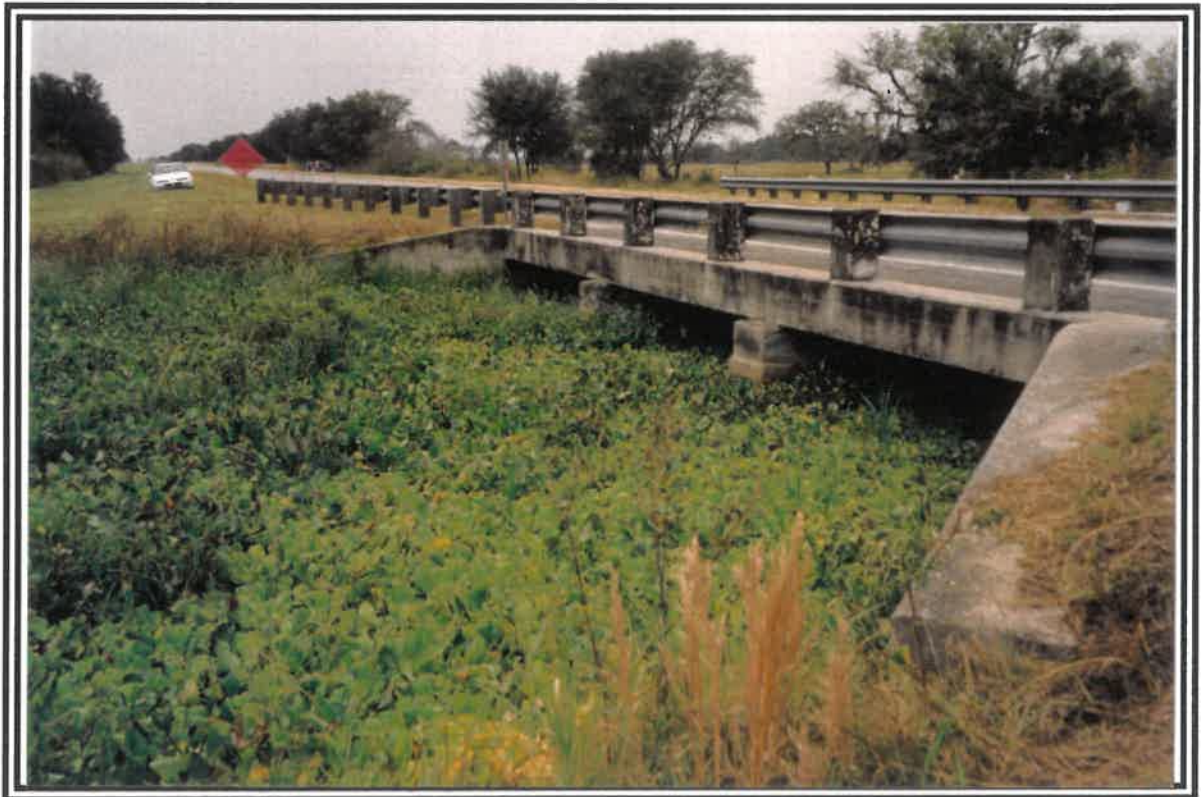
Figure A-5: View South from NE Corner of Bridge (Downstream Side)
