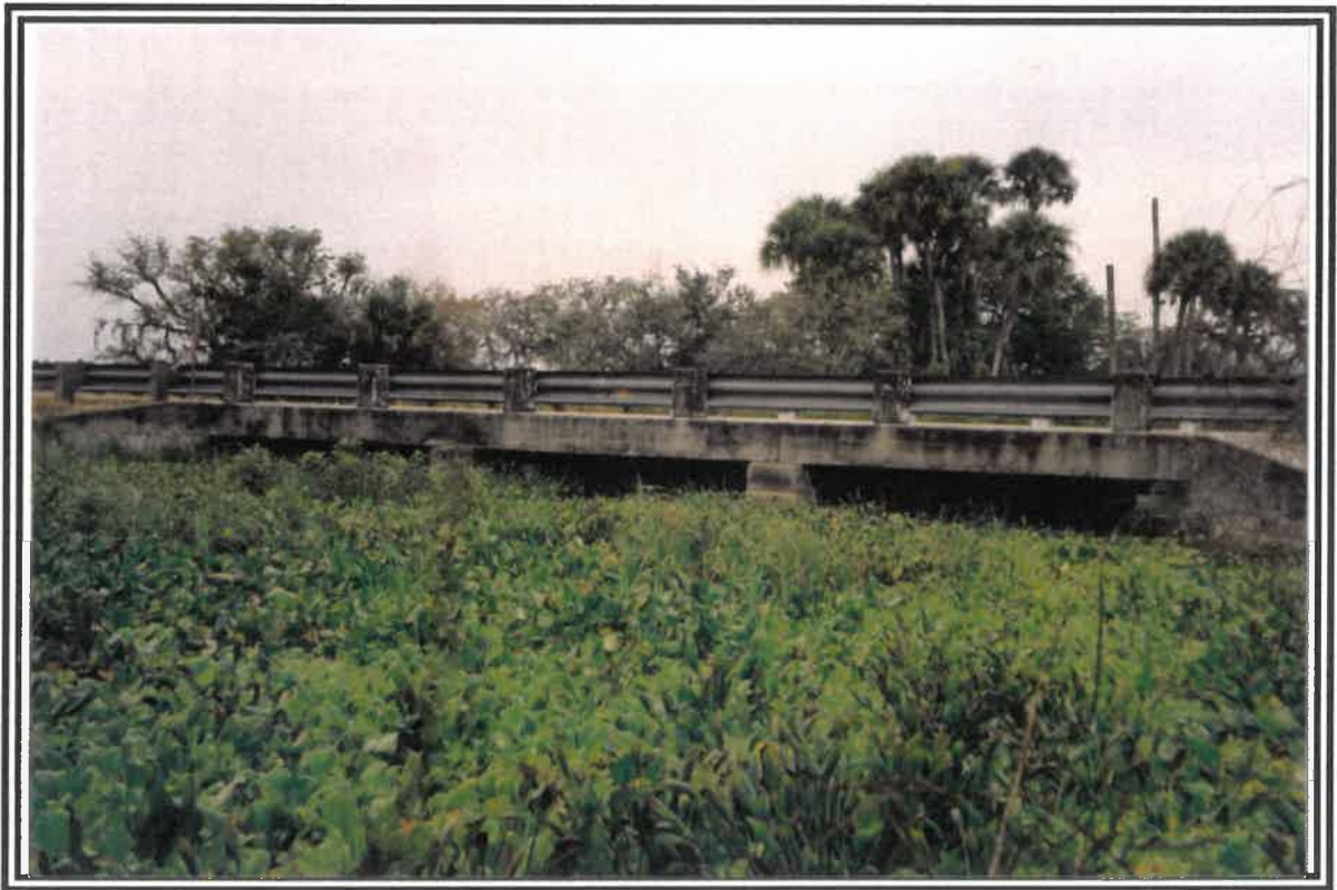
Figure A-1: Bridge No. 050035, Downstream Elevation
