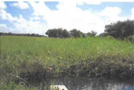
Ditch on northeast side of cross drain.
