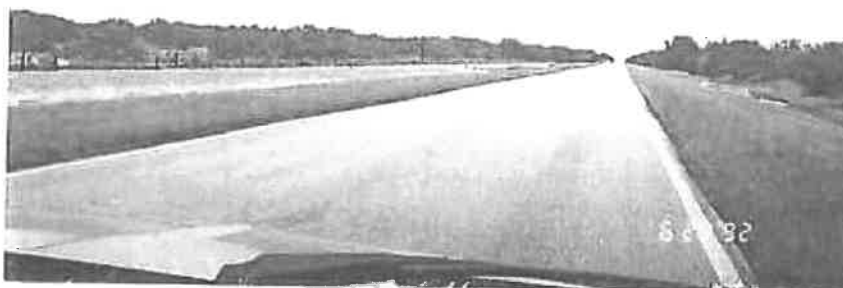
SR 29 - Between Bridge 050033 and SR 78 on June 29, 1992 - wet season.
