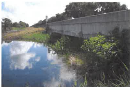
West side of bridge.
