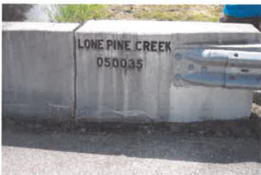
Bridge structure number and name of water body.
