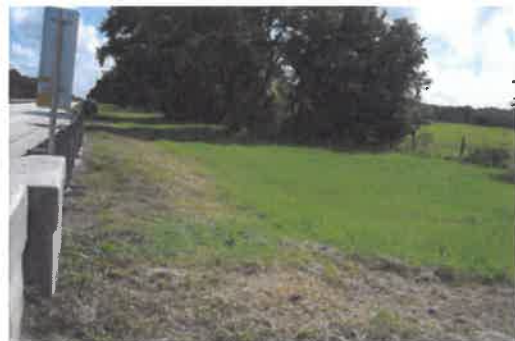
Ditch on northeast side of bridge.
