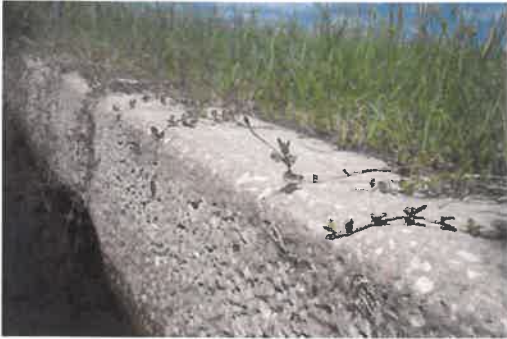
Headwall on east side of cross drain.
