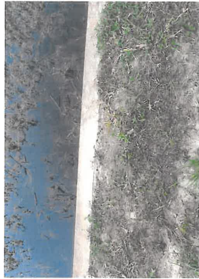
SR 29 Cross Drains (mp 5.50 and 6.257) Glades
