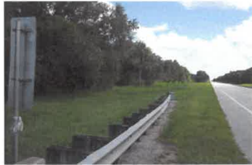
Ditch on northwest side of bridge.
