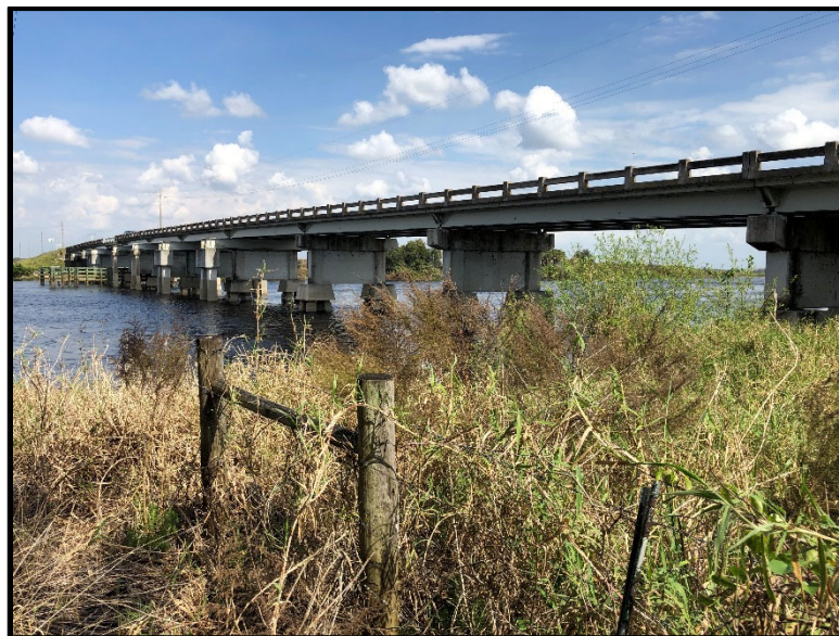
Photo 4 – Photo of acoustic survey Site 2 showing acoustic survey deployment location near the southwest portion of the US 98 bridge.
