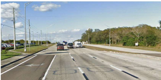
End Project MP 15.286 Southbound
