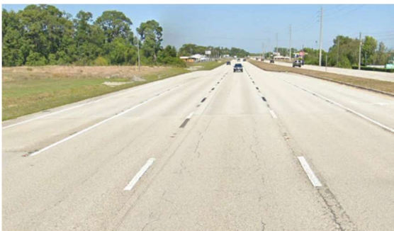
Begin Project MP 11.612 Southbound
