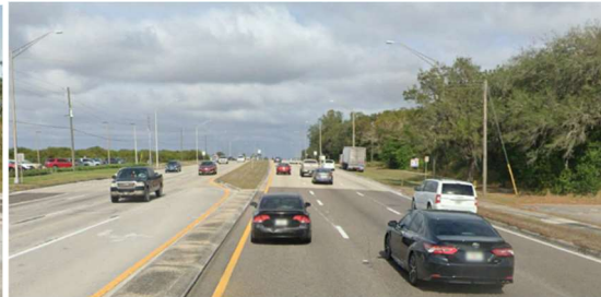
End Project MP 15.286 Northbound
