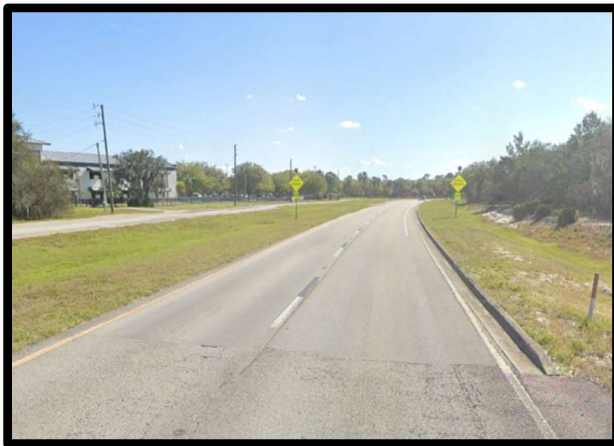
Begin Project MP 6.270
