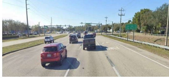
End Project MP 27.030 (SB Pavement Looking SB)
