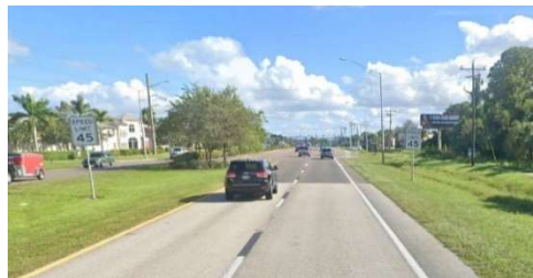
Begin Project MP 25.906 (SB Pavement Looking SB)
