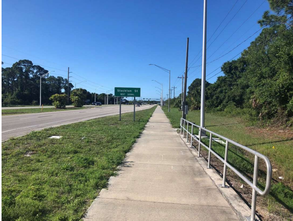
Figure 2: Existing Sidewalk with a Drop-Off Condition and a Pedestrian/Bicycle Railing
