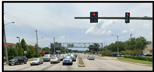
SR 544 at 8 th St NW (US 17) looking west. End Project - MP 3.176
