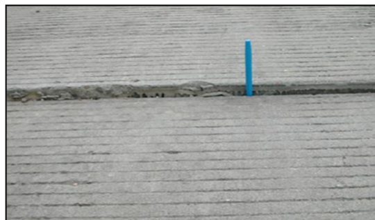
Figure 8: Faulting
