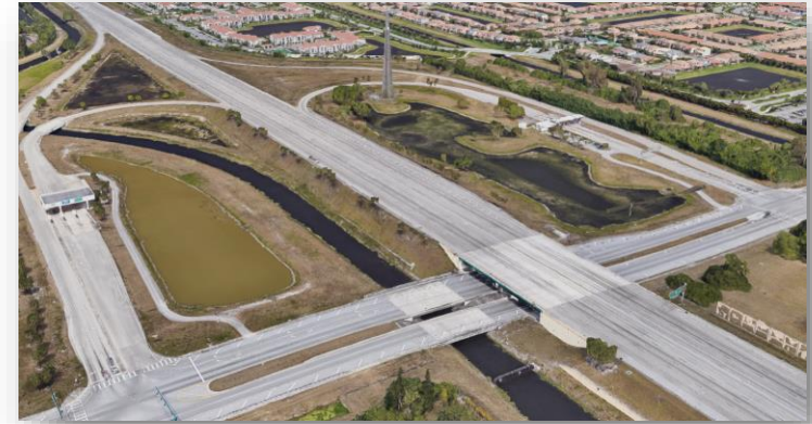
Florida's Turnpike at Atlantic Avenue
