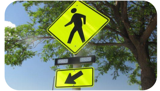
Rectangular Rapid Flashing Beacon
