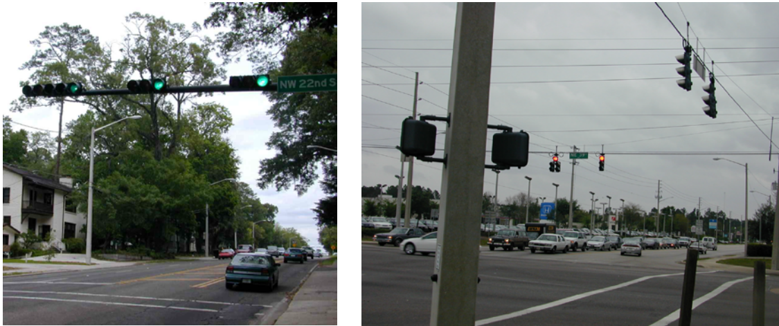
Figure 4-10 Typical Horizontal and Vertical Signal Installations
