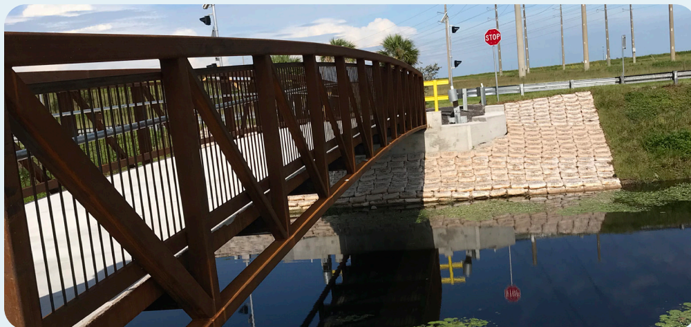
Figure 3: Village of Wellington Pedestrian Bridge at Binks Pointe
