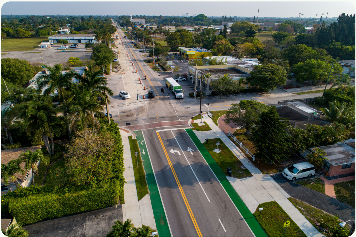
Figure 30: City of Delray Beach Seacrest Boulevard Reconstruction
