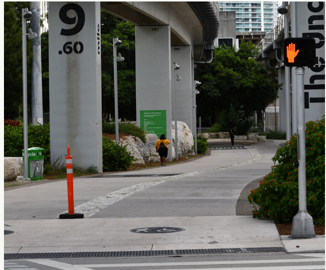
Figure 34: City of Miami Underline Trail
