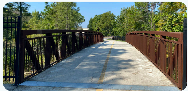
Figure 31: Shingle Creek Regional Trail, prefabricated bridge
