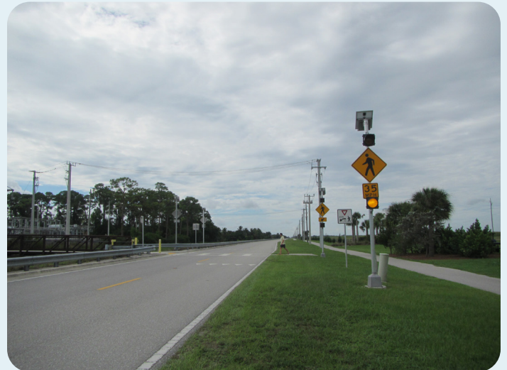
Figure 4: Midblock crossing of Flying Cow Road, Wellington
