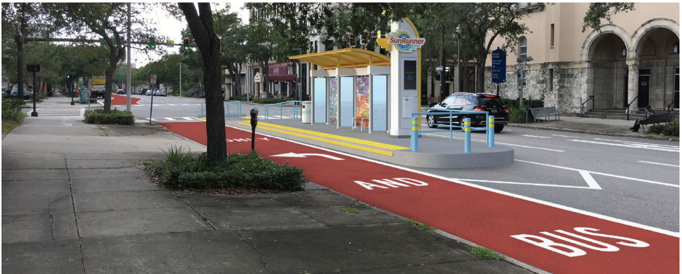
Figure 4-6 Special Use Transit Lanes (PSTA SunRunner rendering shows the BAT lanes that allow turning traffic to utilize the MTL, Pinellas County, FL) Source: PSTA
