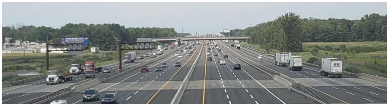
Figure 4-4 Truck-Only Lane Example (Dualized Section of the New Jersey Turnpike)
