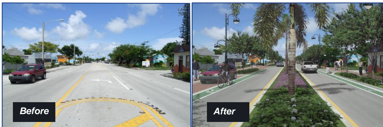
Figure 1: Example Before and After Lane Repurposing
