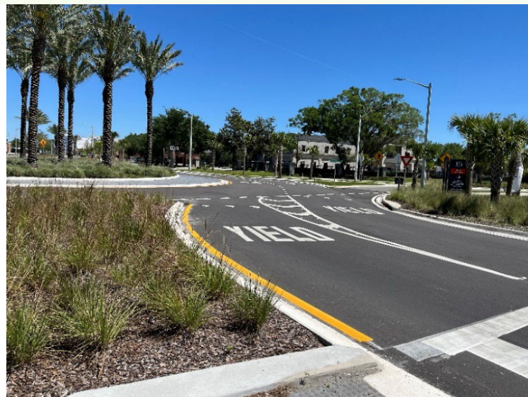
Princeton Street at Texas Avenue roundabout.
