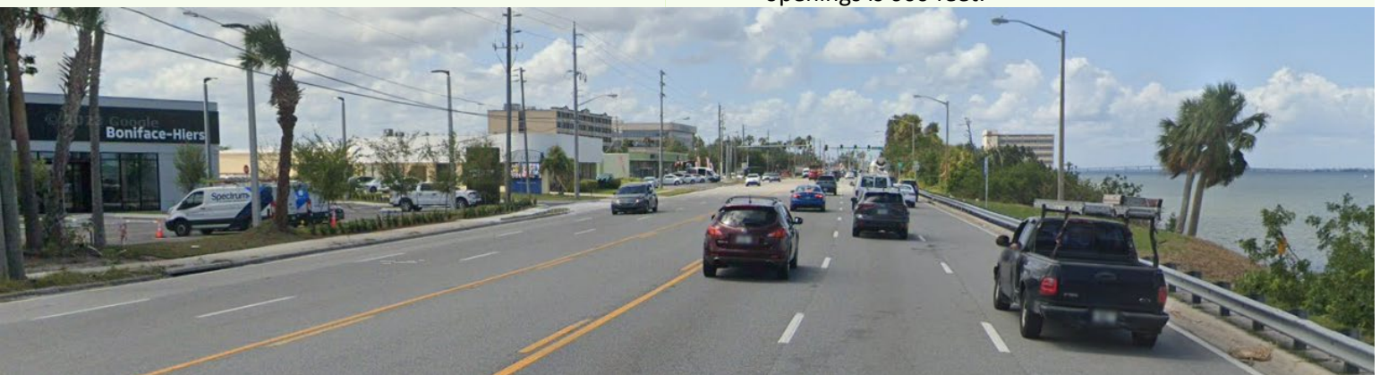
Current US 1 Cross-section in central portion of the corridor.
