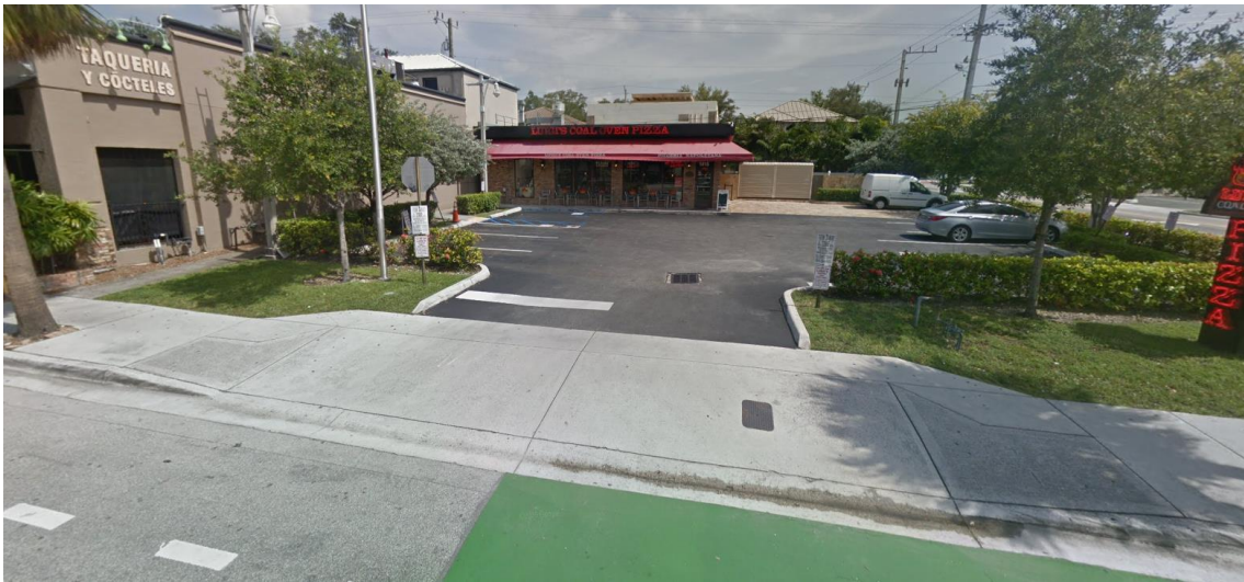
Figure 11 | Curbed Roadway (Flared Return)
