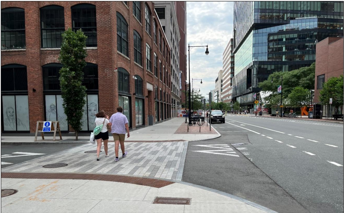
Figure 60 | Raised Sidewalk Crossing
