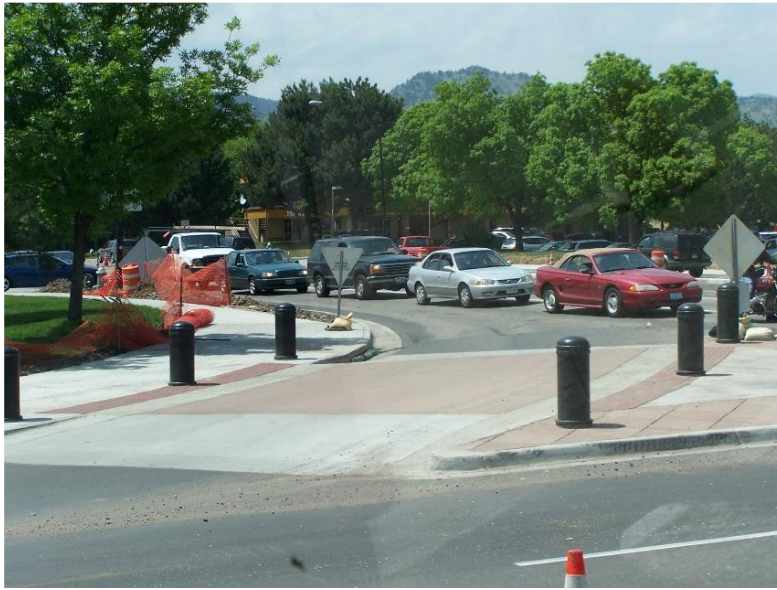
Figure 77 | Raised Crosswalk at Channelized Right Turn
