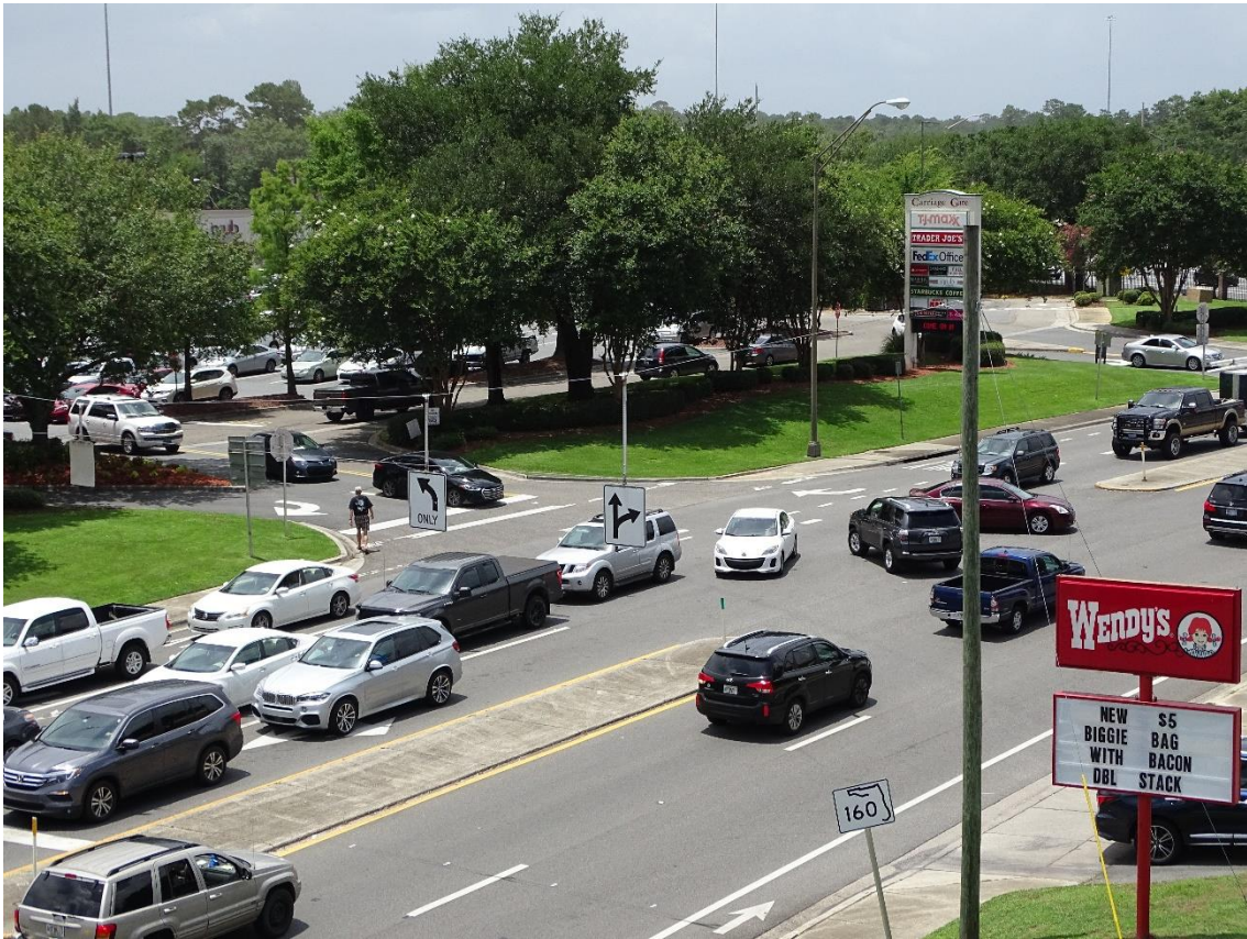
Figure 40 | Vehicles Stopped in Excessively Wide Median Opening
