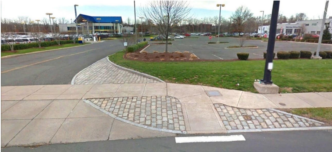
Figure 105 | Truck Apron and Driveways
