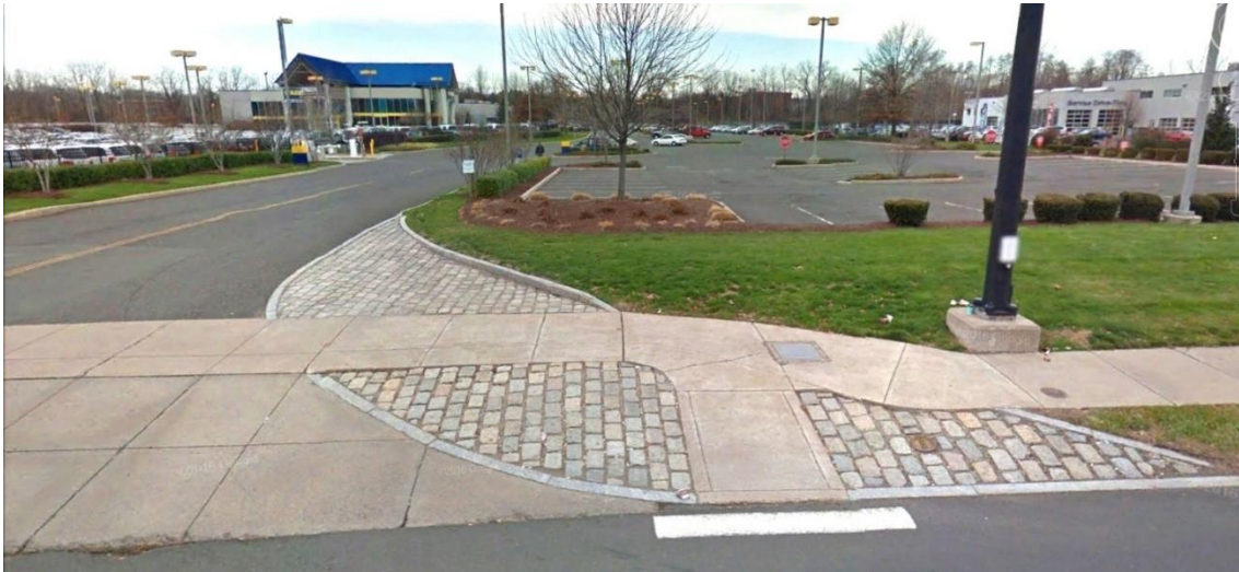
Figure 87 – Truck Apron and Driveways
