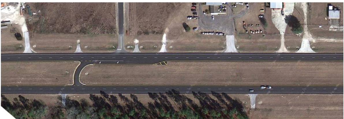
Figure 70 – Truck U-Turn in Williston, FL
