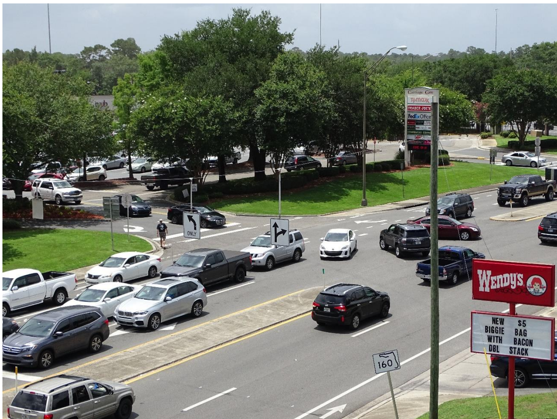
Figure 31 – Vehicles Stopped in Excessively Wide Median Opening
