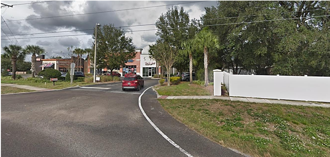
Figure 5 – Flush Shoulder Roadway (Radial Return)
