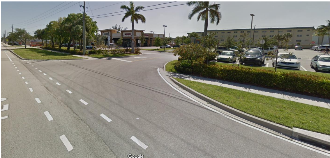
Figure 6 – Curbed Roadway (Radial Return)
