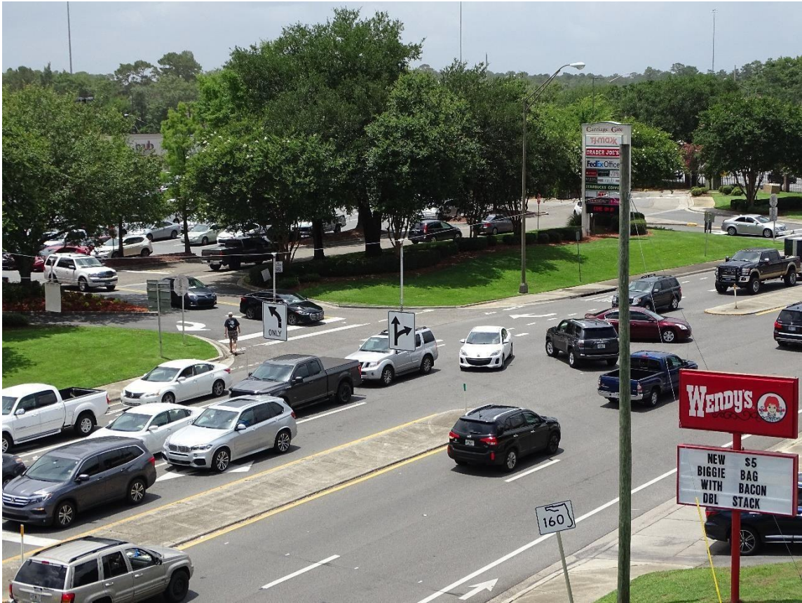
Figure 40 | Vehicles Stopped in Excessively Wide Median Opening
