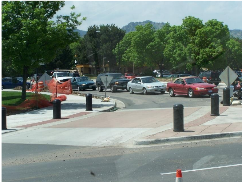
Figure 77 | Raised Crosswalk at Channelized Right Turn
