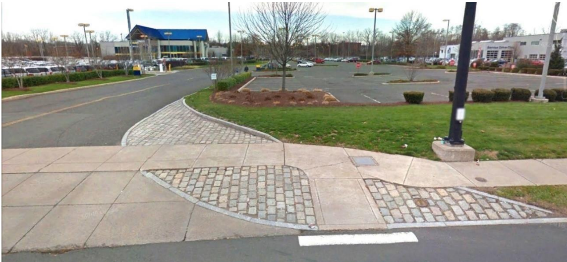
Figure 105 | Truck Apron and Driveways
