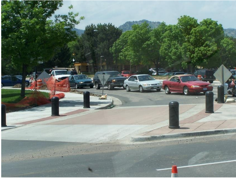
Figure 77 | Raised Crosswalk at Channelized Right Turn
