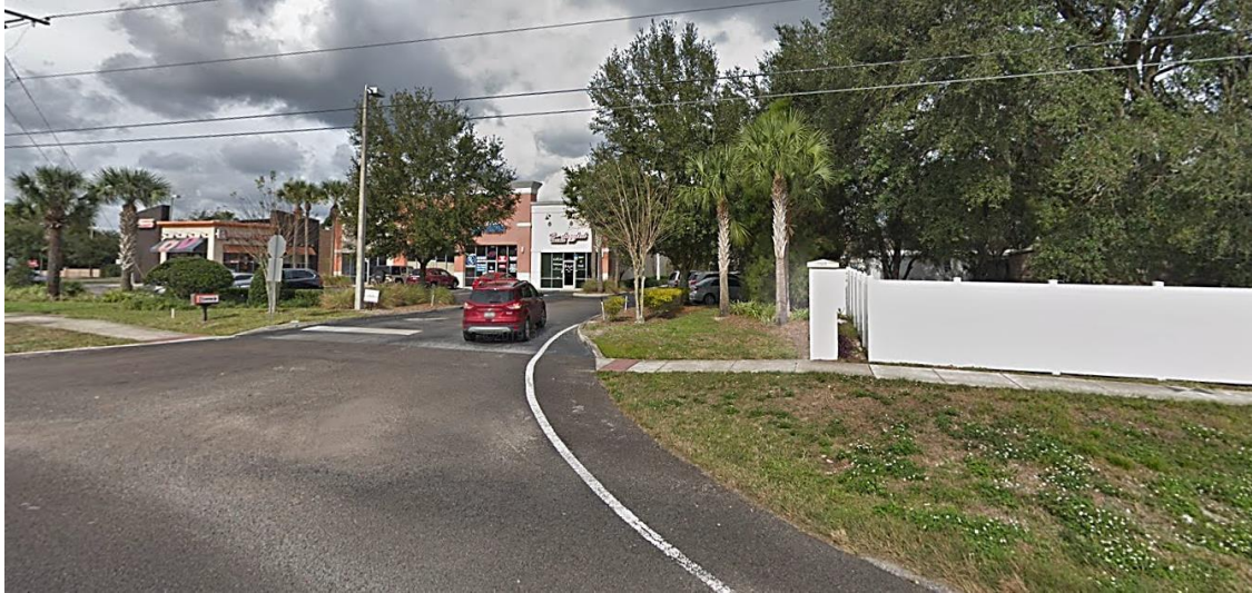
Figure 9 | Flush Shoulder Roadway (Radial Return)
