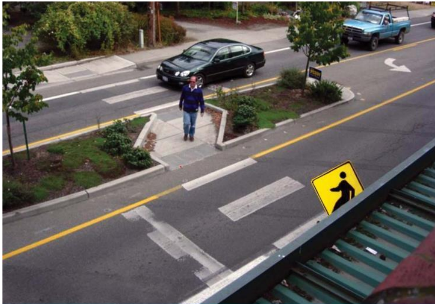
Figure 100 | Angled Pedestrian Refuge Crossing
