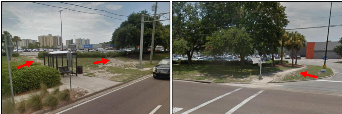
Figure 94 | Worn Footpaths between Bus Stop, Crosswalk, and Major Retail Center
