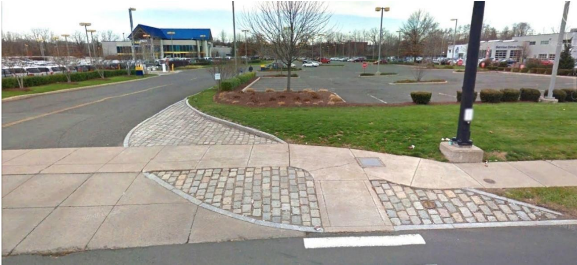
Figure 105 | Truck Apron and Driveways
