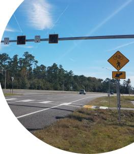
The pedestrian hybrid beacon, mounted on a mast arm, is designed to alert motorists and help trail visitors safely cross State Road 207
