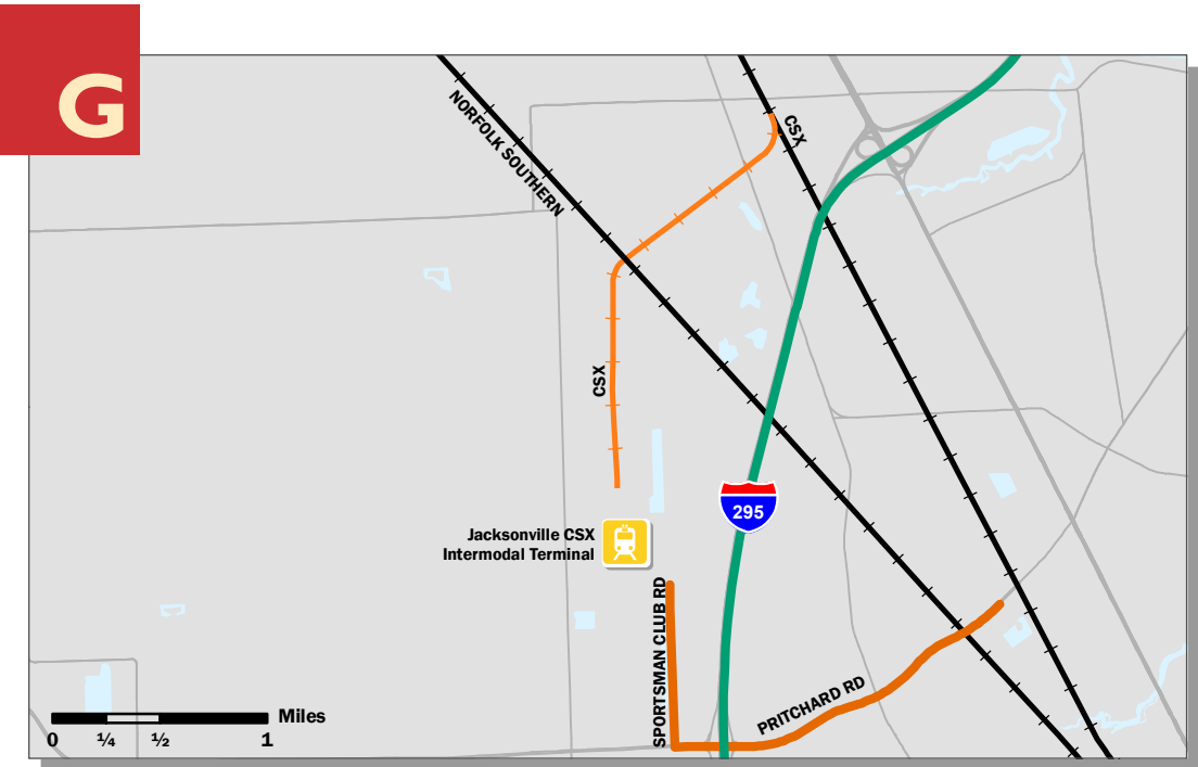
Jacksonville CSX Intermodal Terminal
