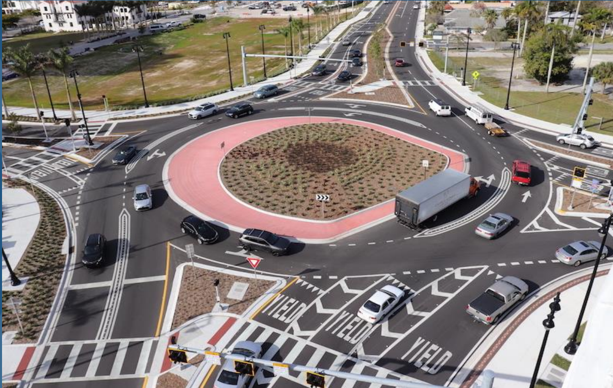
US 41 Roundabout Corridor, City of Sarasota
