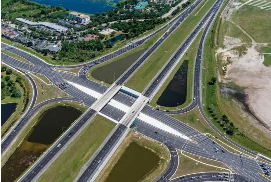
Image 1. Diverging Diamond Interchange in Sarasota, Florida (Google Earth)
