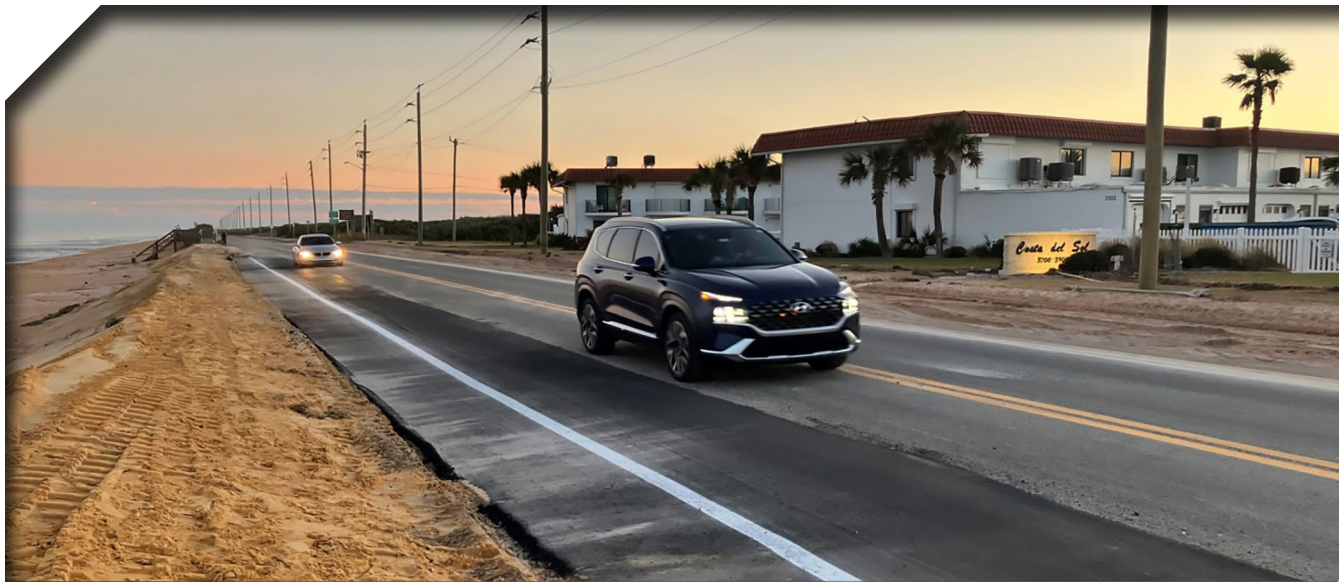
SR A1A repairs following Hurricane Nicole
