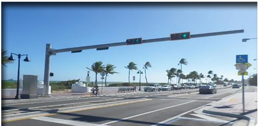
SR A1A resilience improvements following Hurricane Sandy, Ft. Lauderdale
