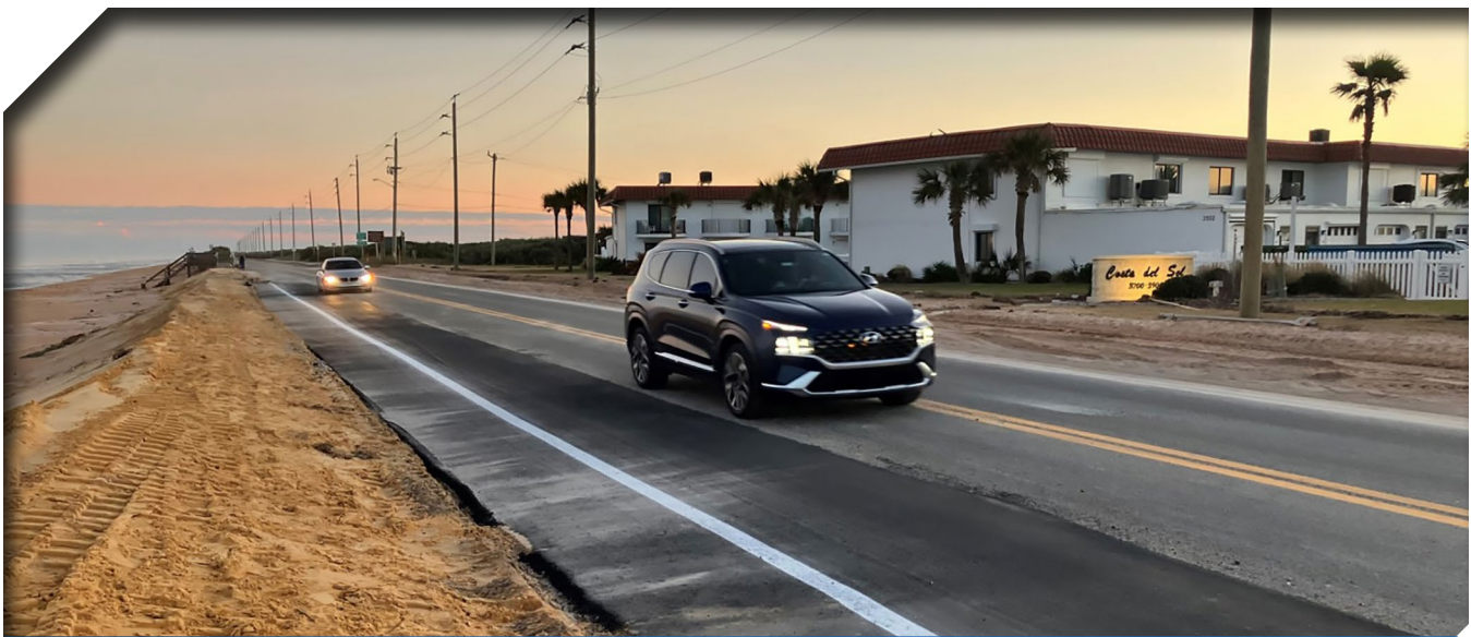
SR A1A repairs following Hurricane Nicole
