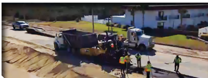
SR A1A emergency repair after Hurricane Nicole, Flagler County
