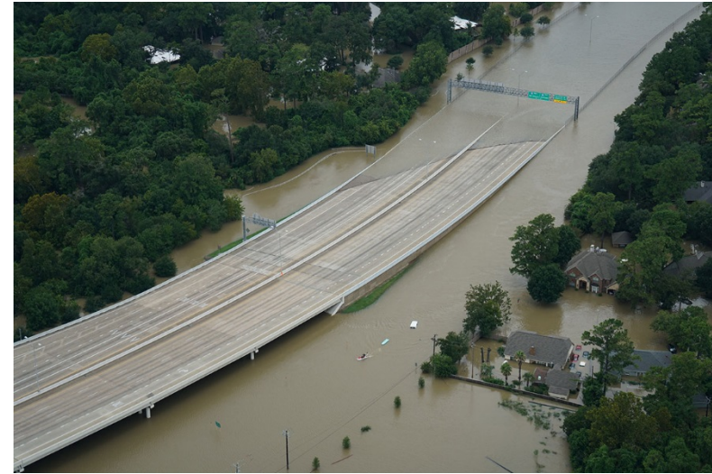
Flooding from Hurricane Harvey, Credit: TTI
