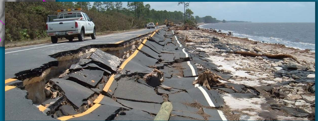
US 98 in Franklin County. FDOT
