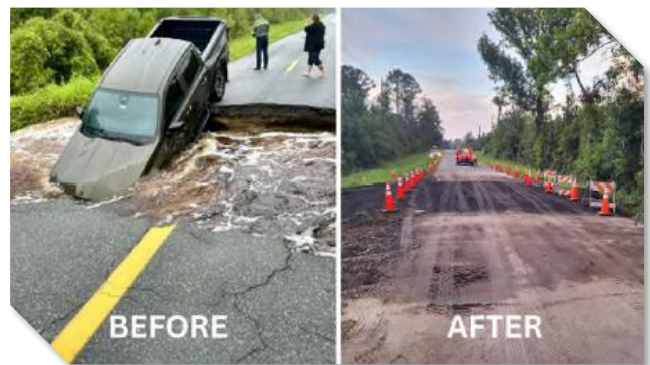
Road Repair for Hurricane Debby (2024)
