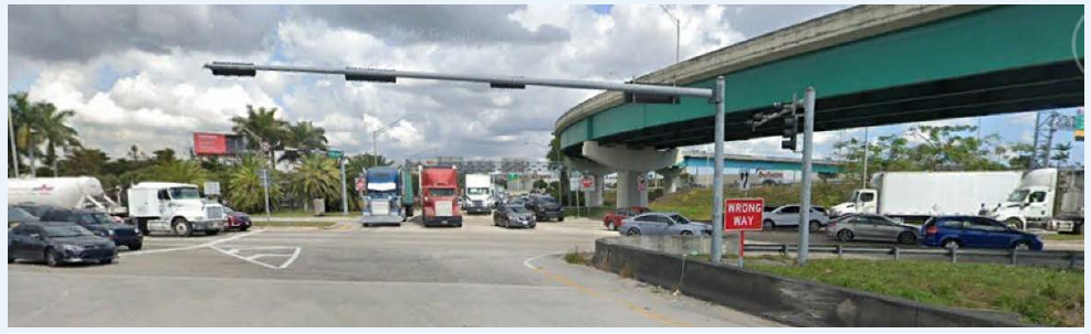
Okeechobee Road looking west at SR 826 / Palmetto Expressway
