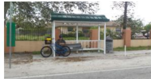
These transit facilities that do have sidewalks adjacent to them do not adhere to ADA criteria.
