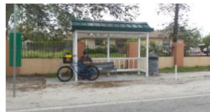
These transit facilities that do have sidewalks adjacent to them do not adhere to ADA criteria.
