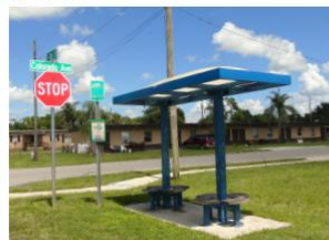
Most of the bus stops in Immokalee do not have sidewalks or bikeways that connect to them.
