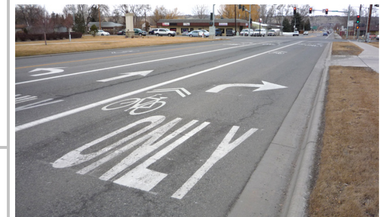
Combined Bike Lane/Turn Lane with Shared Lane Markings in Billings, MT
