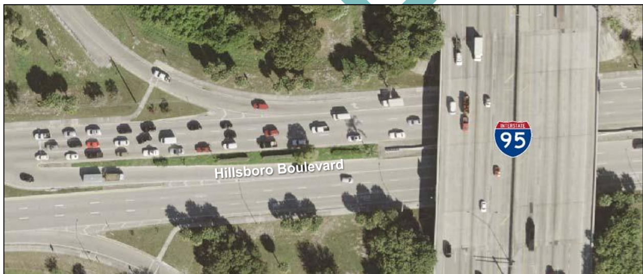
Figure 3 - 5: Existing Roadway Segment – Hillsboro Boulevard
