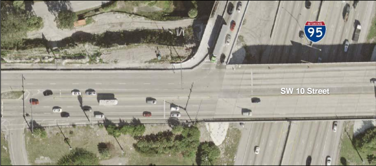
Figure 3 - 3: Existing Roadway Segment – SW 10 th Street
