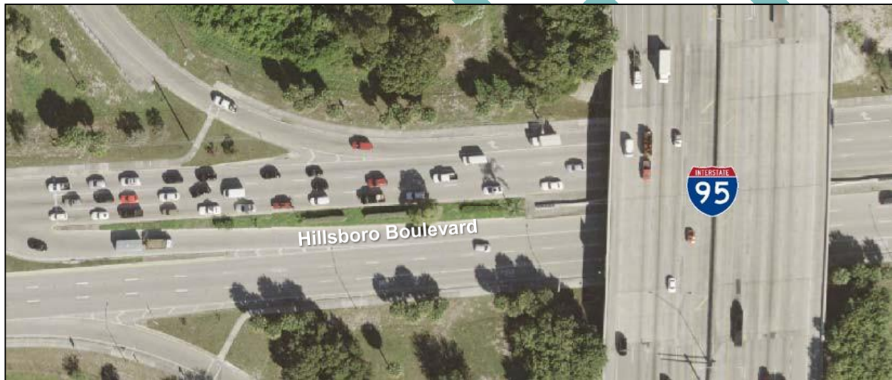
Figure 3 - 5: Existing Roadway Segment – Hillsboro Boulevard
