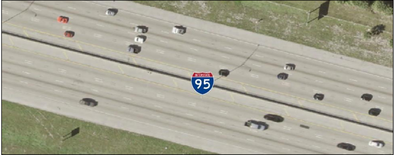
Figure 3 - 1: Existing Roadway Segment – I-95 Corridor
