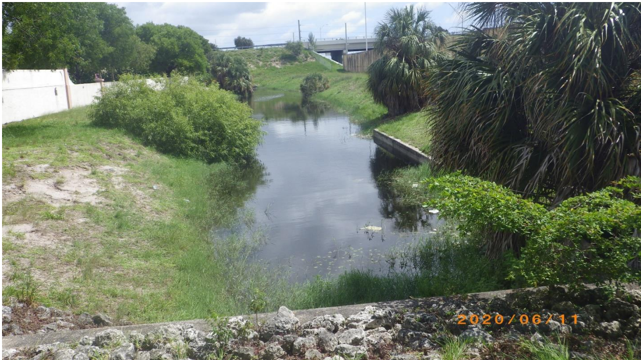
Photo 12: Surface Water 11 – facing north from south culvert FLUCFCS – 534 / FWS – POWHx
