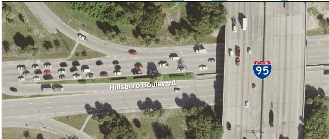
Figure 3 - 5: Existing Roadway Segment – Hillsboro Boulevard
