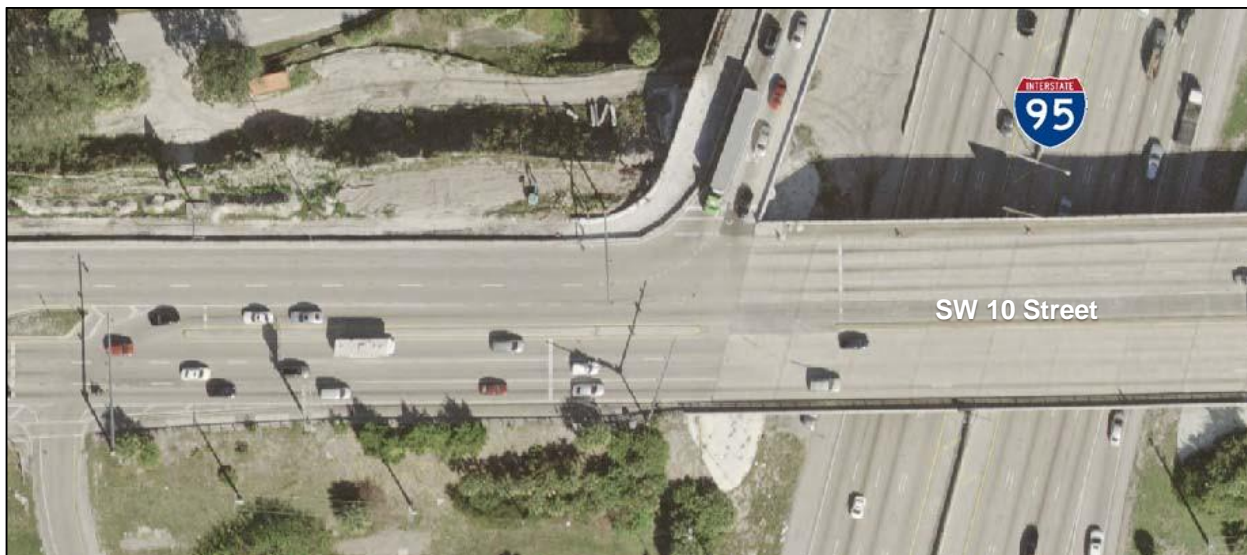
Figure 3 - 3: Existing Roadway Segment – SW 10 th Street
