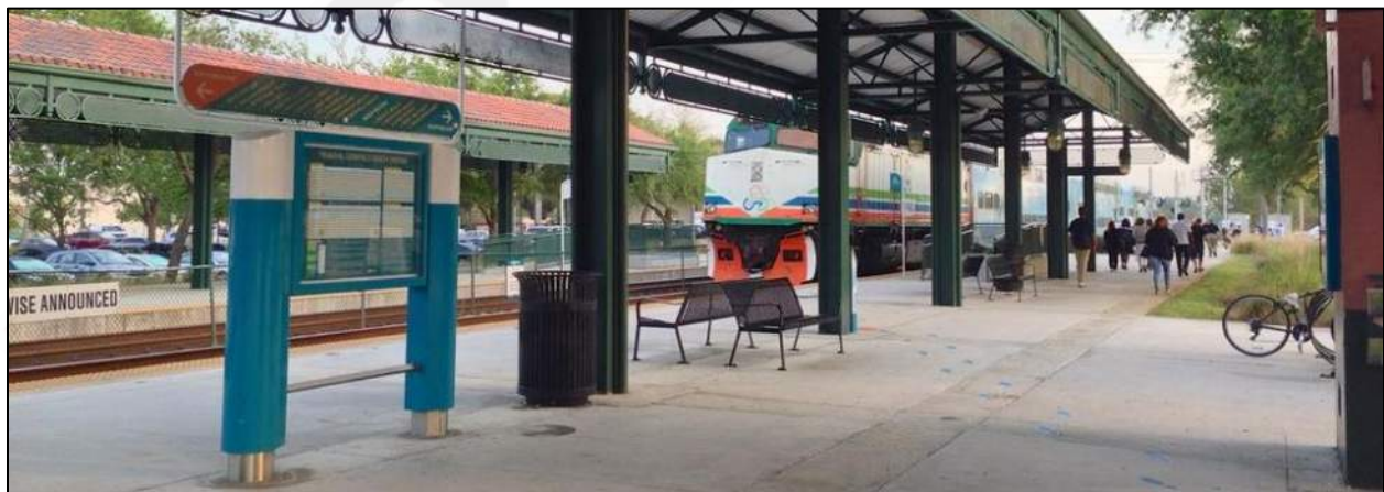
Figure 2-20 Deerfield Beach Station
