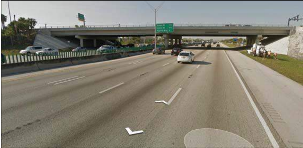
Figure 2-14 Bridge No. 860123 Looking South
