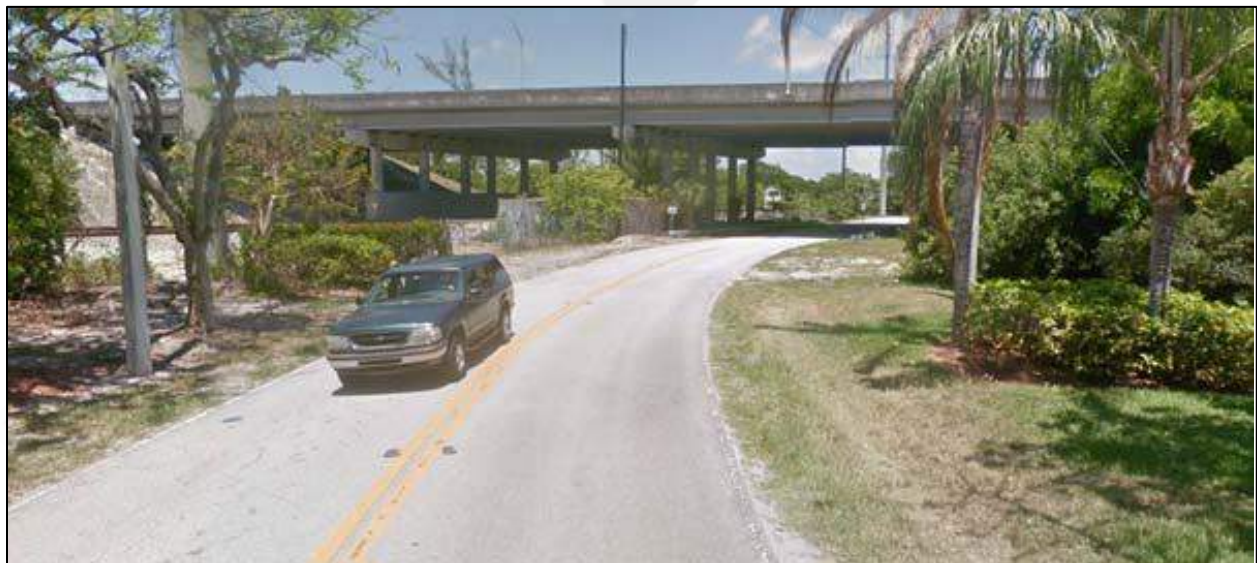
Figure 2-17 Bridge No. 860557 Looking North
