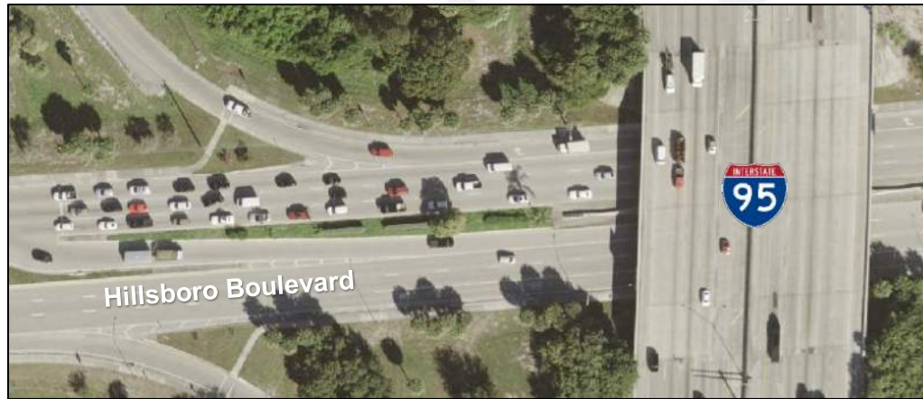
Figure 2-5 Existing Roadway Segment – Hillsboro Boulevard
