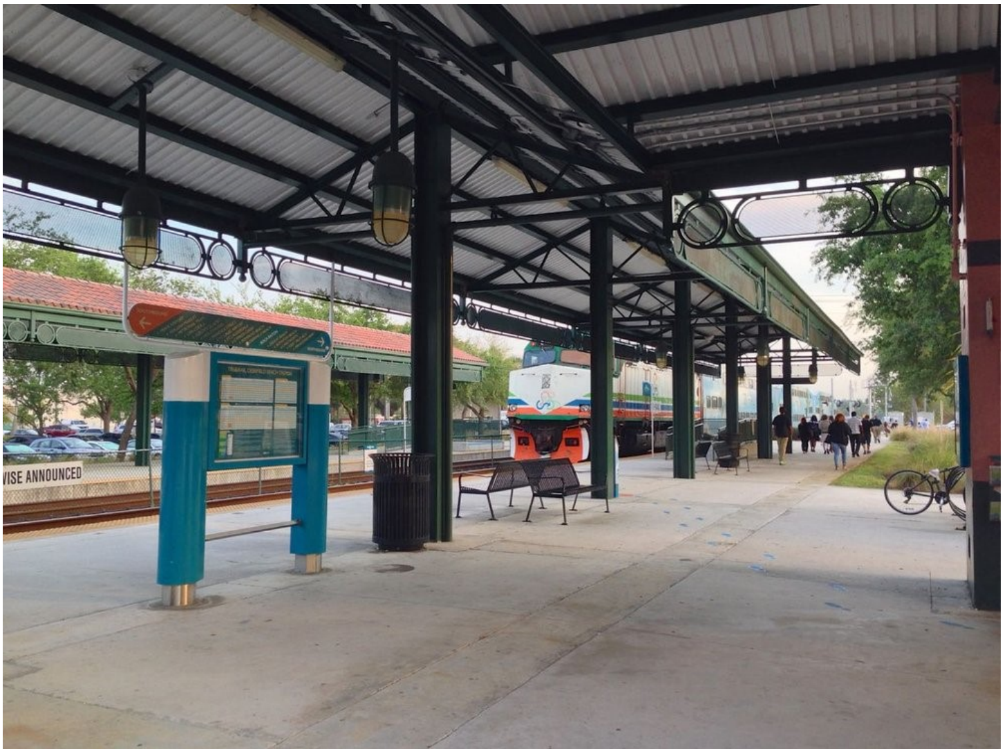
Figure 1 - 9: Deerfield Beach Station
