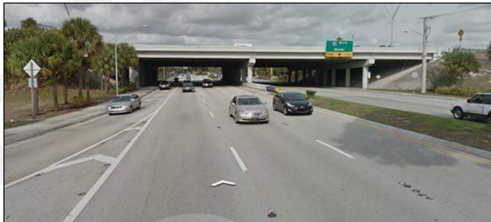
Figure 2-10 Bridge No. 860194 Looking West
