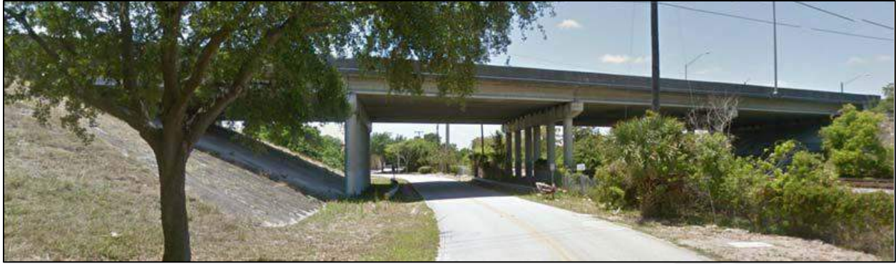
Figure 2-18 Bridge No. 860553 Looking South
