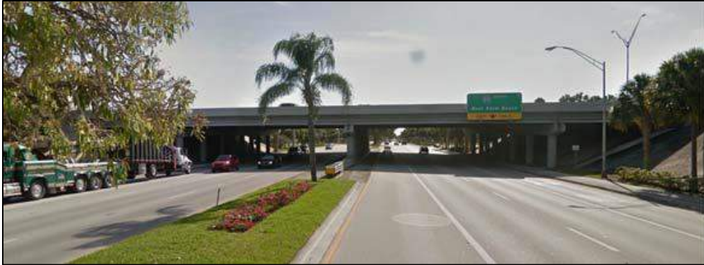
Figure 2-11 Bridge No. 860124 Looking East
