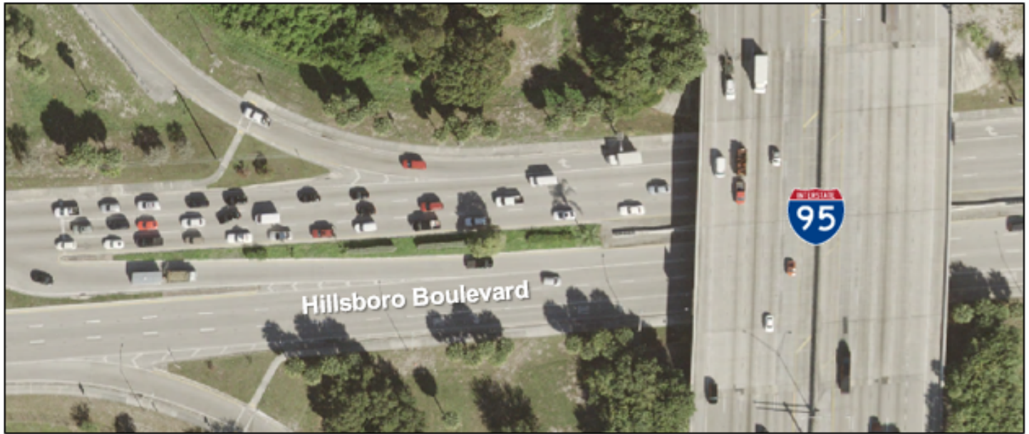
Figure 1 - 6: Existing Roadway Segment - Hillsboro Boulevard
