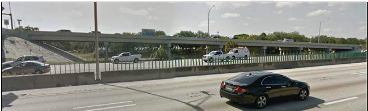
Figure 2-15 Bridge No. 860564 Looking West
