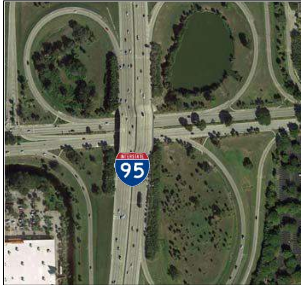
Figure 2-9 Bridges at Hillsboro Boulevard and I-95 Interchange (Bridge Nos. 861094 & 860124)
