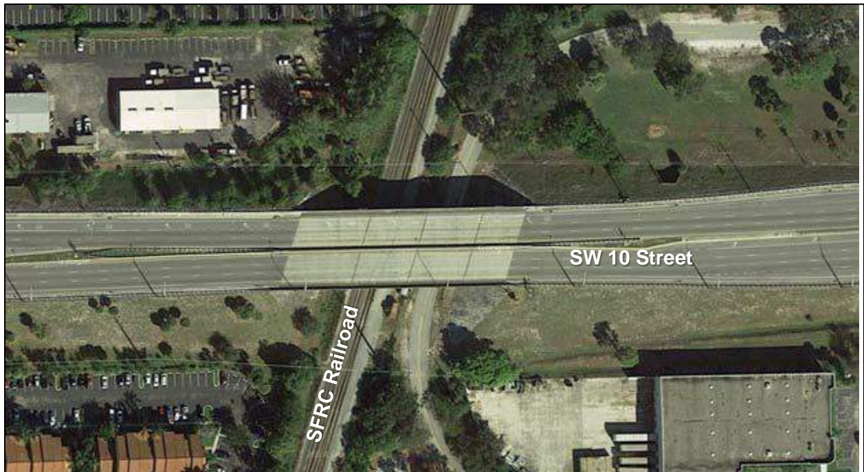
Figure 2-16 Bridges at SW 10 Street and SW 12 Avenue / SFRC Railroad Interchange (Bridge Nos. 860557 & 860553)
