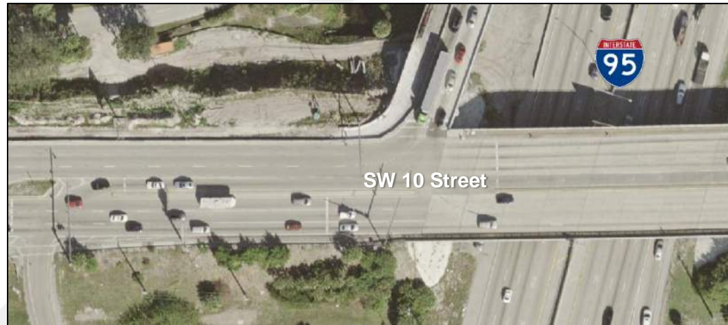
Figure 2-3 Existing Roadway Segment – SW 10 Street
