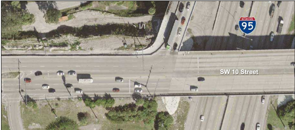
Figure 2-3 Existing Roadway Segment – SW 10th Street
