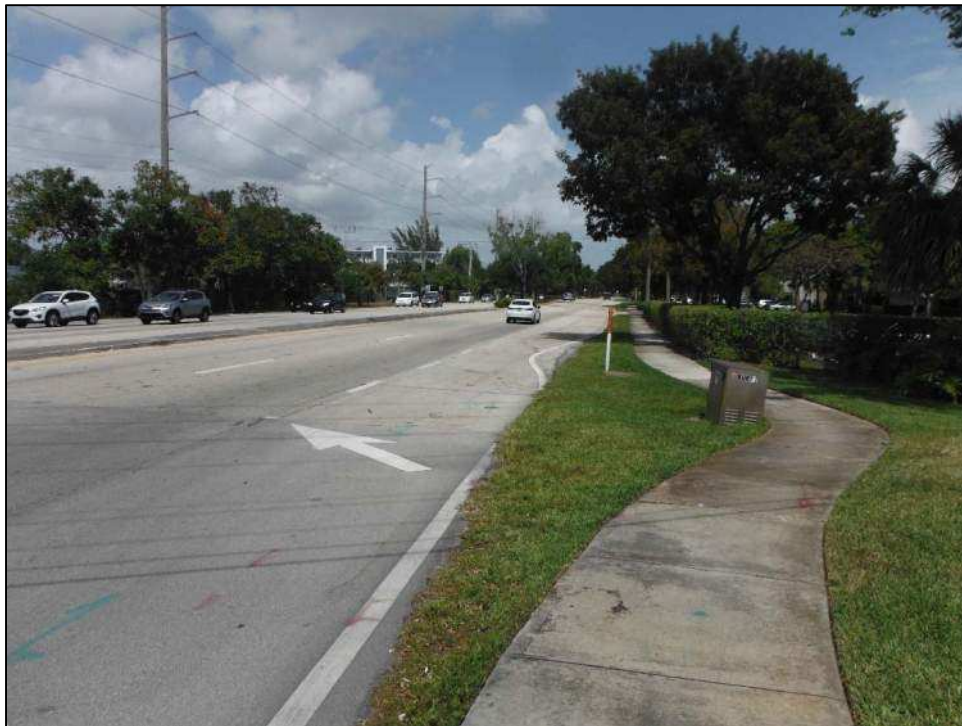
Figure 11-2 Military Trail from SW 10th Street, facing north
