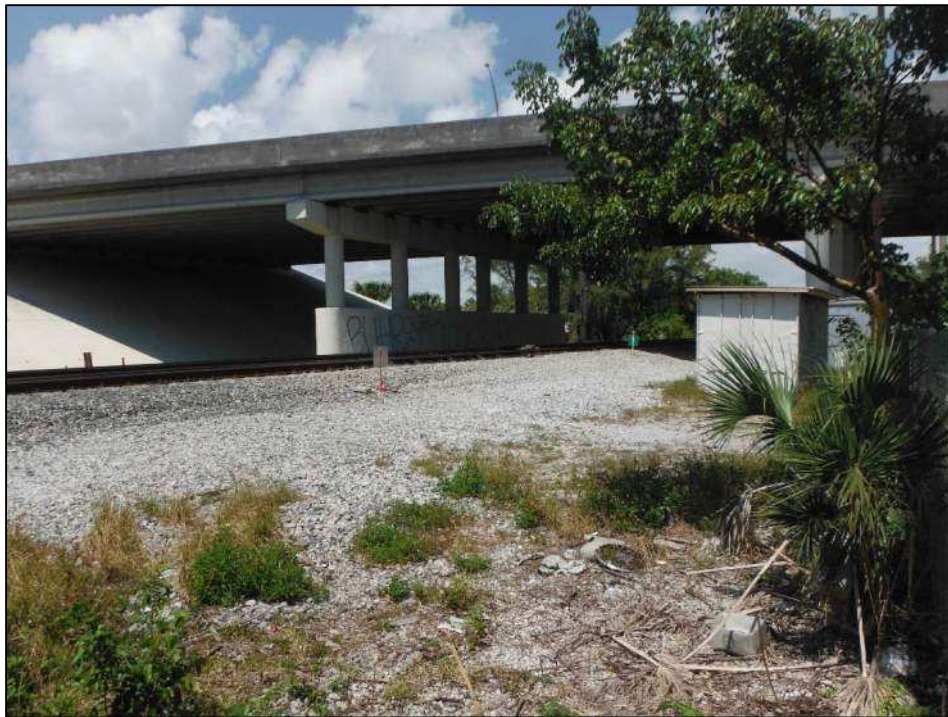
Figure 11-6 Seaboard Air Line (CSX) Railroad (8BD4649) at intersection with SW 10th Street overpass, facing north
