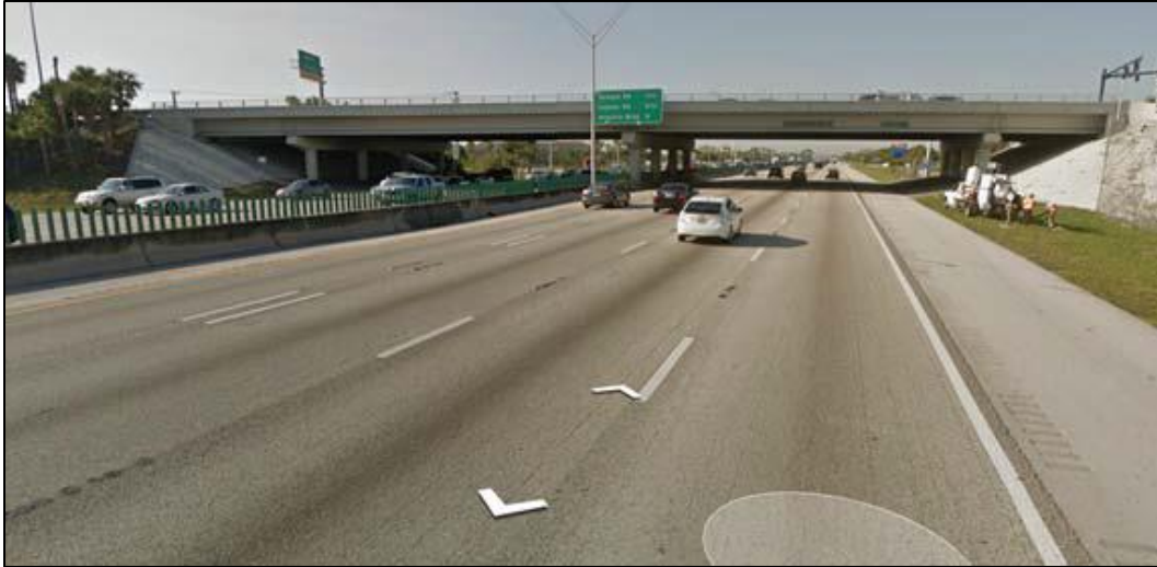
Figure 2-14 Bridge No. 860123 Looking South
