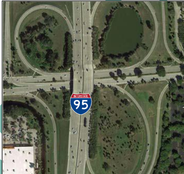
Figure 2-9 Bridges at Hillsboro Boulevard and I-95 Interchange (Bridge Nos. 860194 & 860124)
