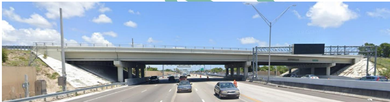
Figure 2-20 Bridge No. 860122 Looking North
