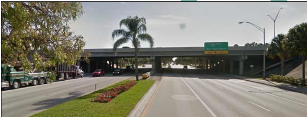
Figure 2-11 Bridge No. 860124 Looking East
