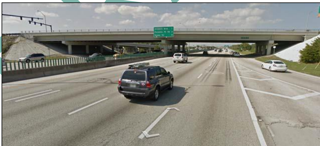
Figure 2-13 Bridge No. 860123 Looking North
