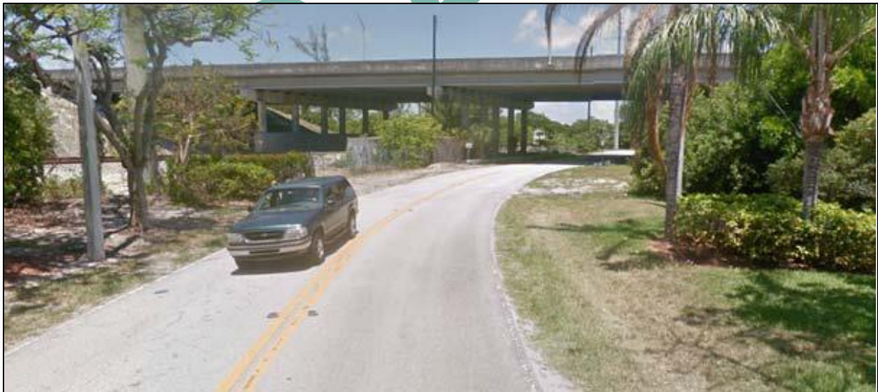
Figure 2-17 Bridge No. 860557 Looking North
