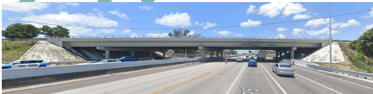
Figure 2-21 Bridge No. 860122 Looking South
