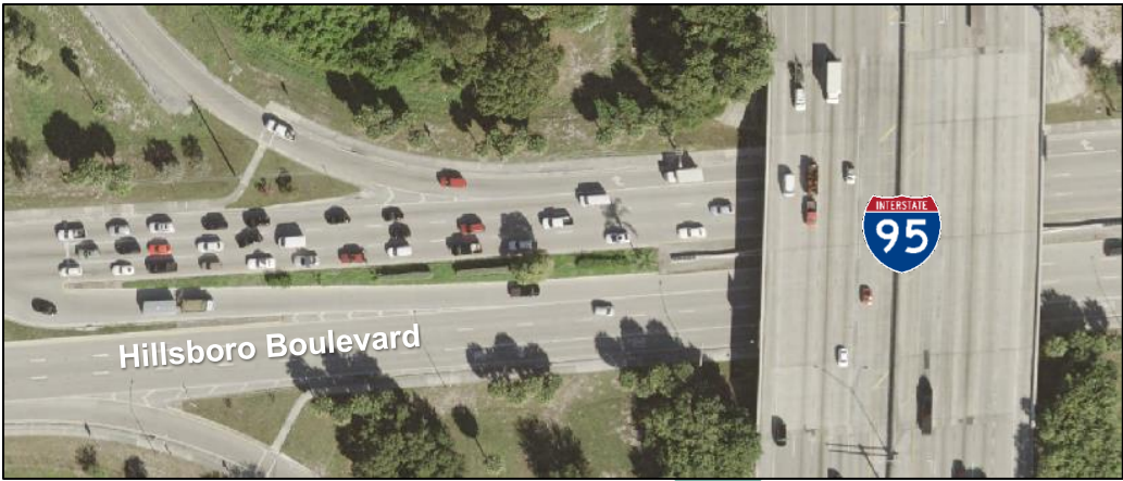
Figure 2-5 Existing Roadway Segment – Hillsboro Boulevard
