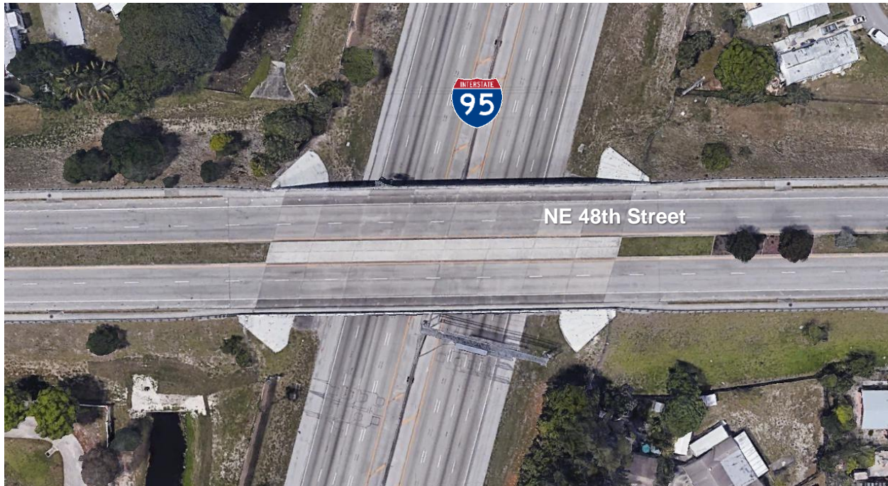
Figure 2-19 NE 48th Street and I-95 (Bridge No. 860122)
