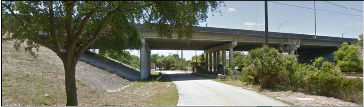
Figure 2-18 Bridge No. 860553 Looking South
