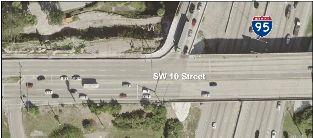
Figure 2-3 Existing Roadway Segment – SW 10 Street
