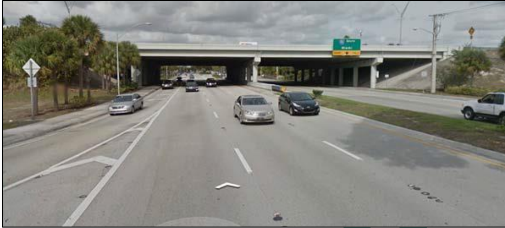
Figure 2-10 Bridge No. 860194 Looking West
