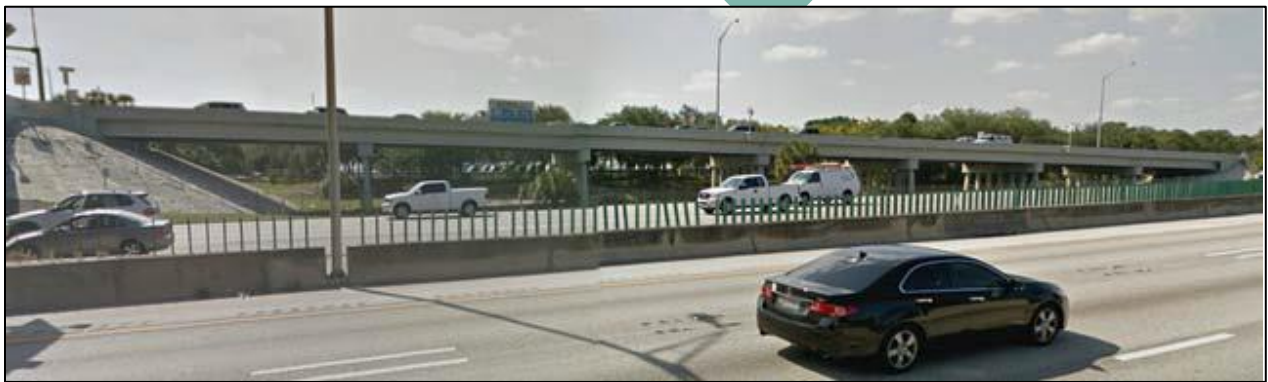
Figure 2-15 Bridge No. 860564 Looking West
