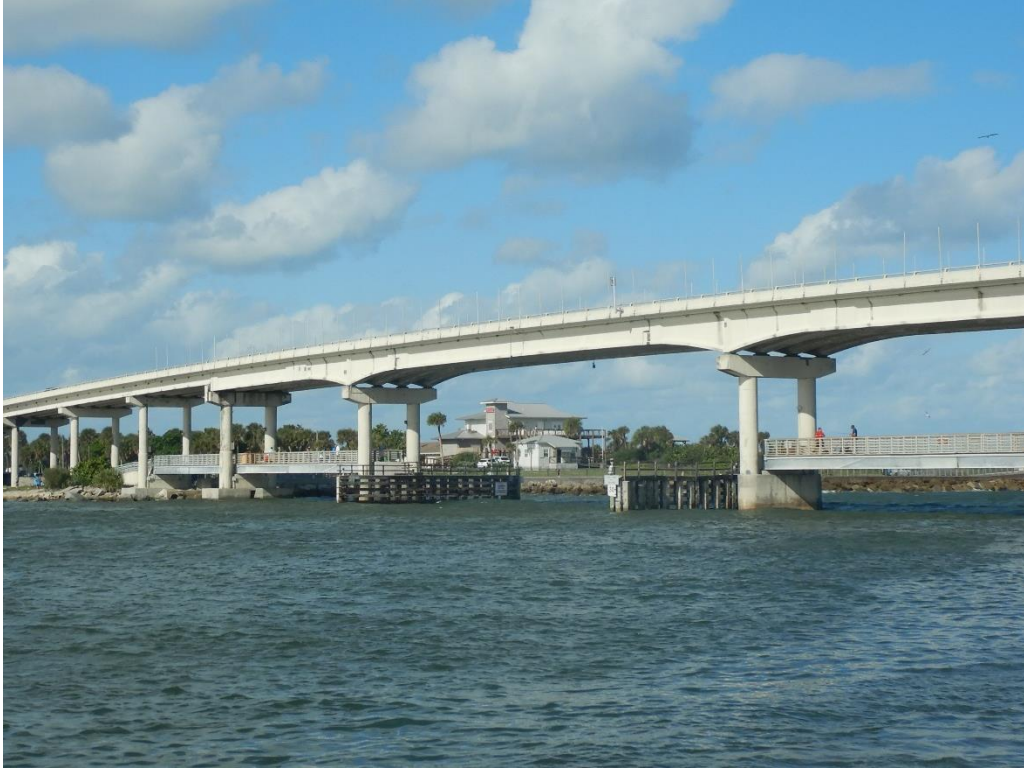
Sebastian Inlet Bridge from the west, facing towards the east.
