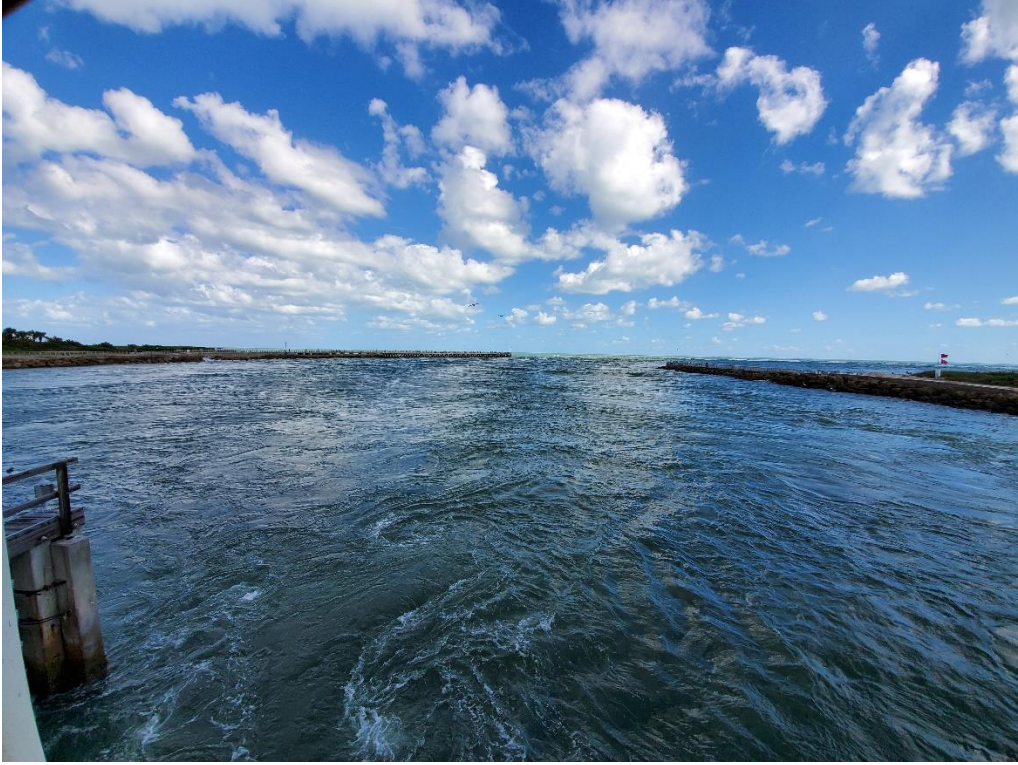
Sebastian Inlet Bridge channel facing towards the east to the Atlantic Ocean
