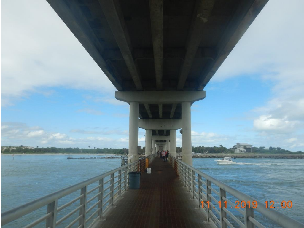
Underdeck of Sebastian Inlet Bridge, facing north along bridge alignment.
